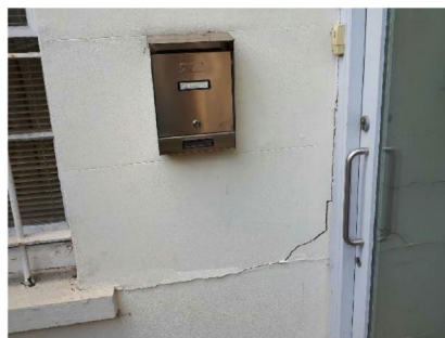
Cracking Adjacent to Basement Door
