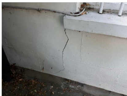
Cracking Below Basement Window
