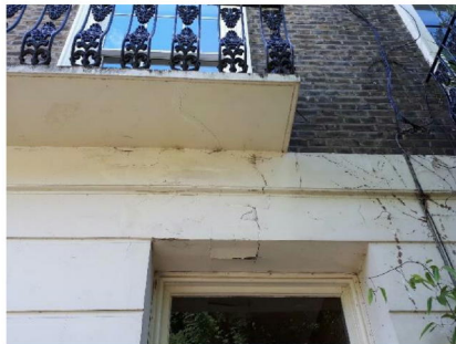
Cracking Above Front Door
