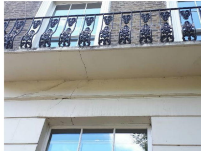
Cracking Above Ground Floor Window
