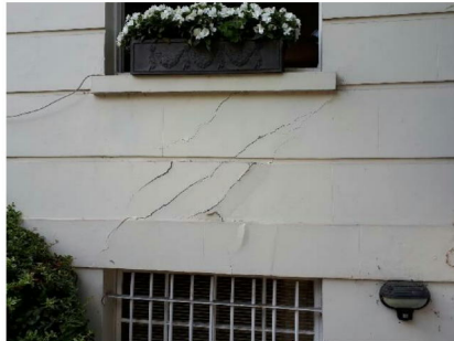
Cracking Above Basement Window
