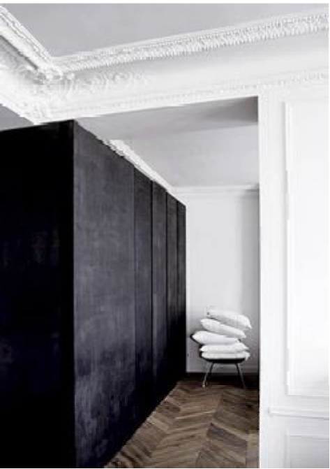
Examples of internal 'pod' treatment (design intent), painted panels (no skirtings), 15mm 'lash-gap' detail at junction with original wall volumes/ party walls and at floors.
