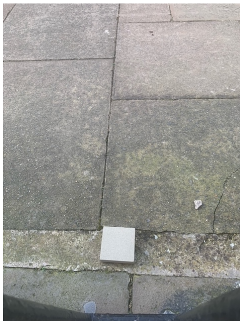
Photo D: Sample of proposed stone on existing misshapen stone tread
