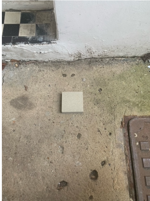
Photo B: Sample of proposed stone on existing lightwell floor finish
