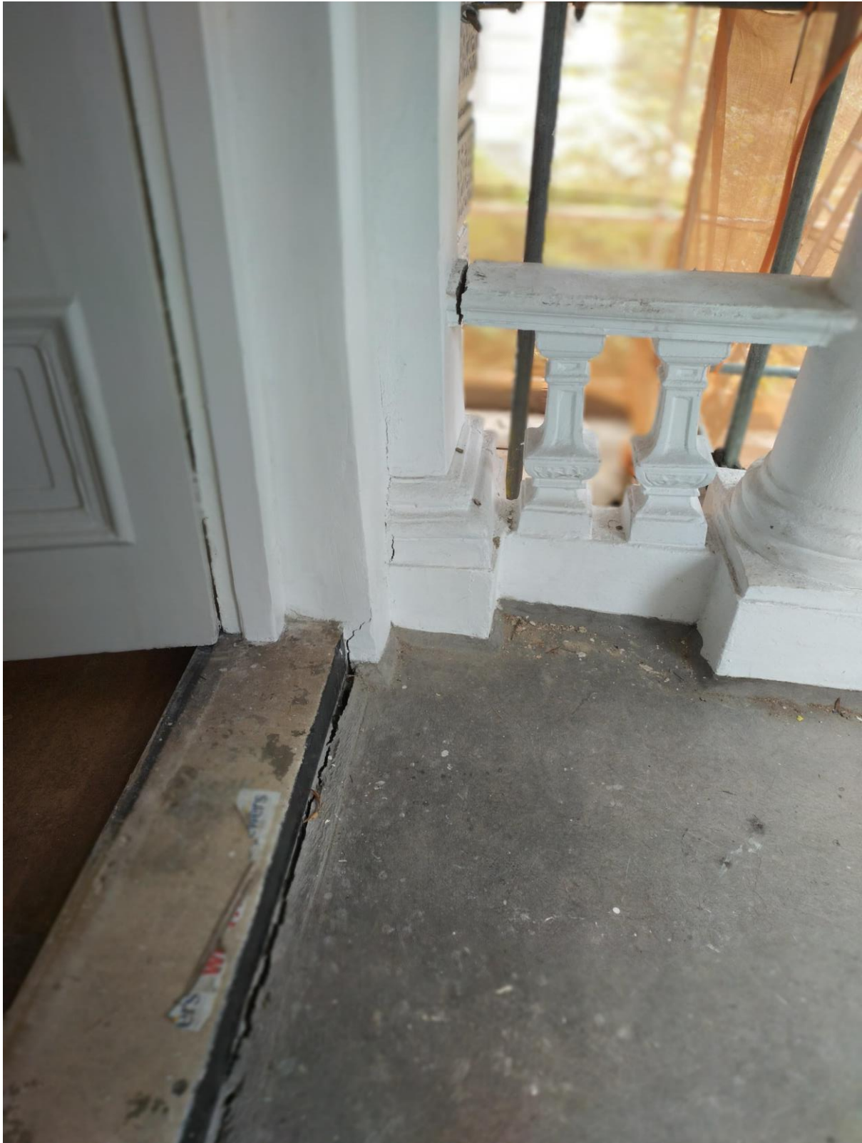
Photo 9 – Step damage
