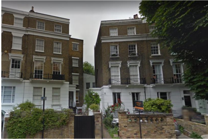
Existing gap between no.29 and 30
