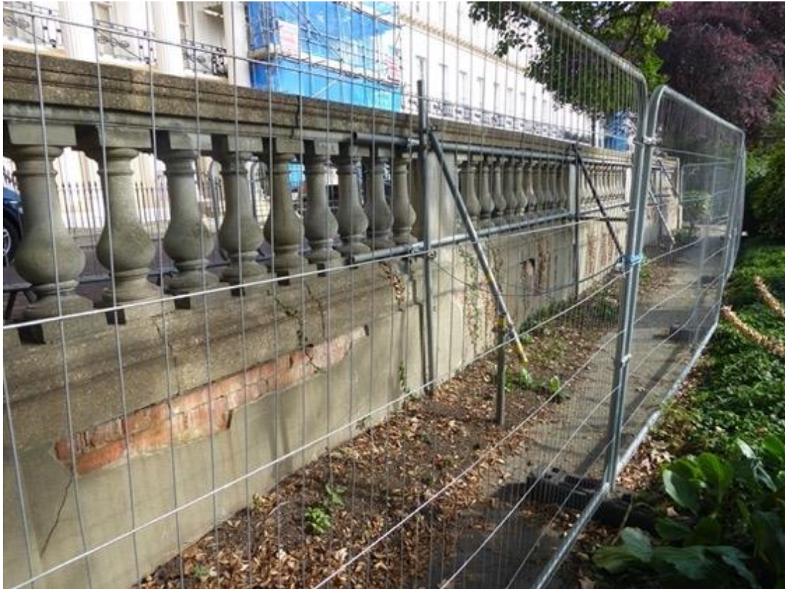
6.View looking south: balustrade showing brick base, fencing and scaffold bracing
