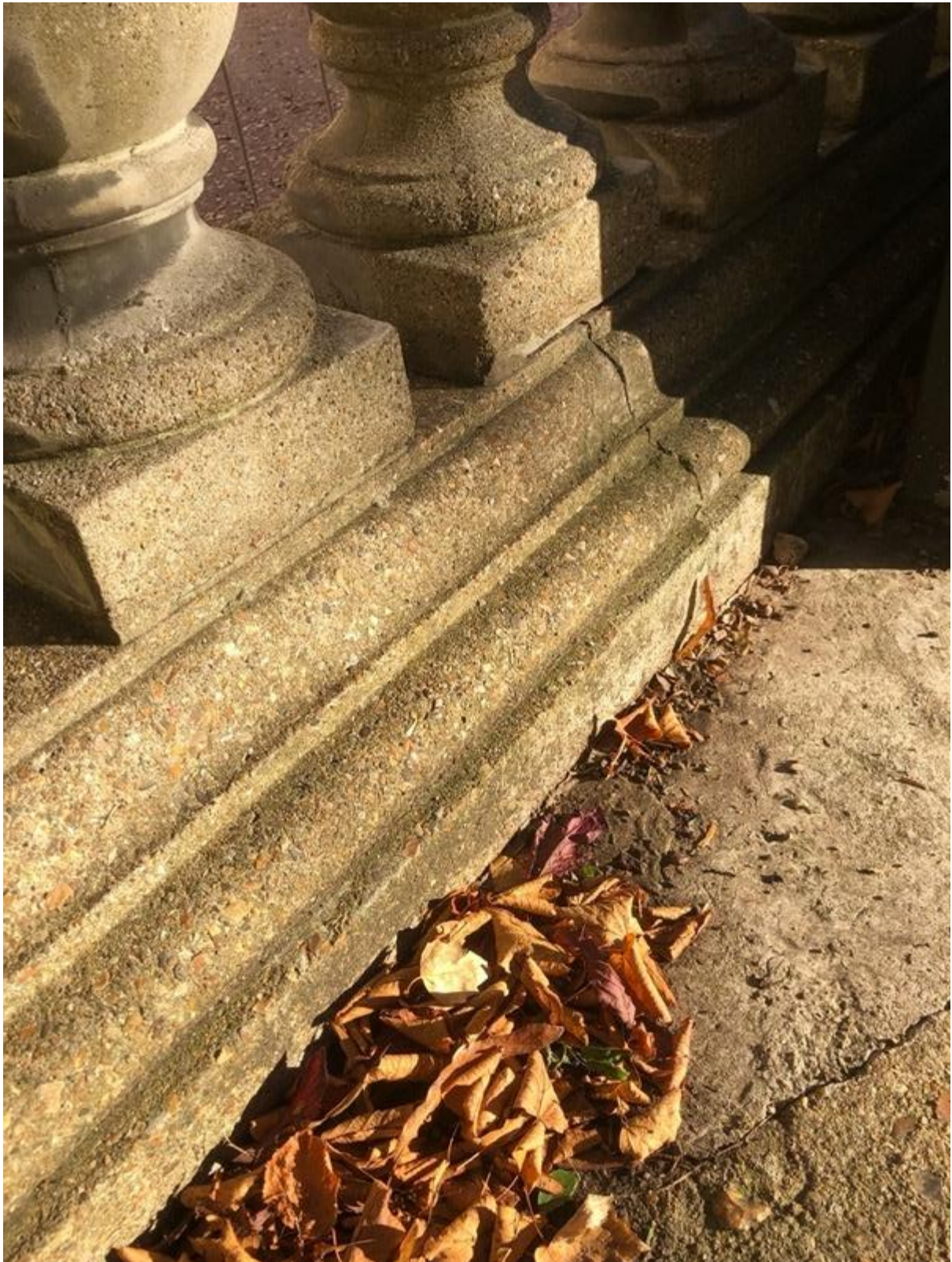
11.Moulded base of balustrade to garden side only
