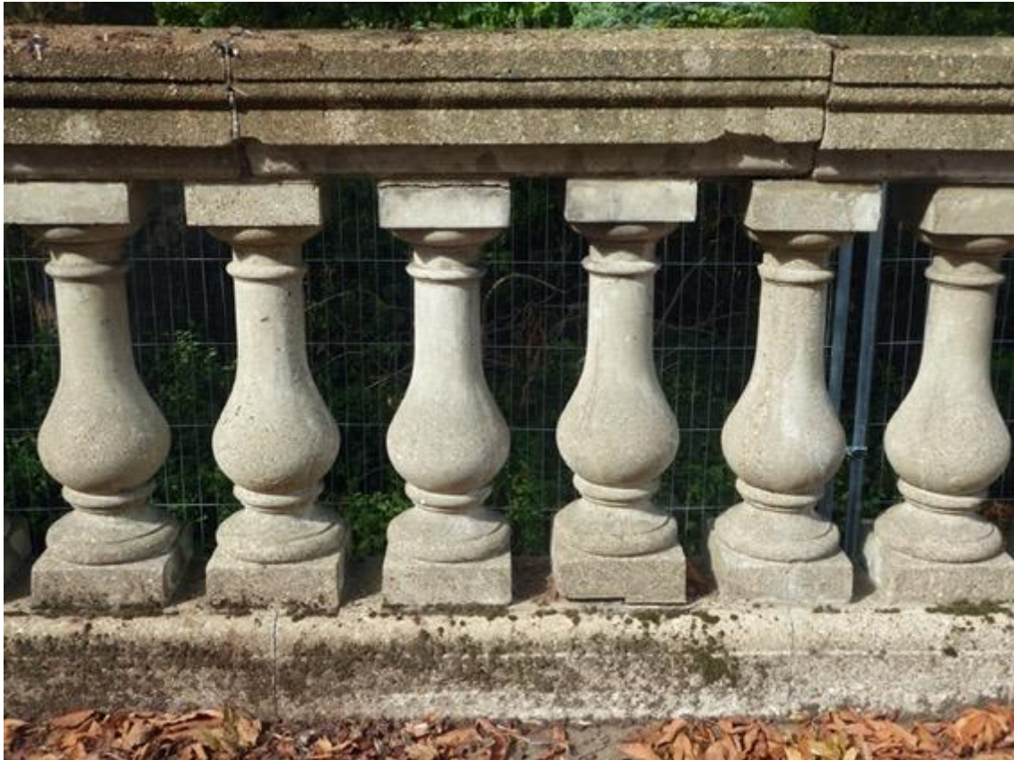
8. Deflected bottle balustrade and capping
