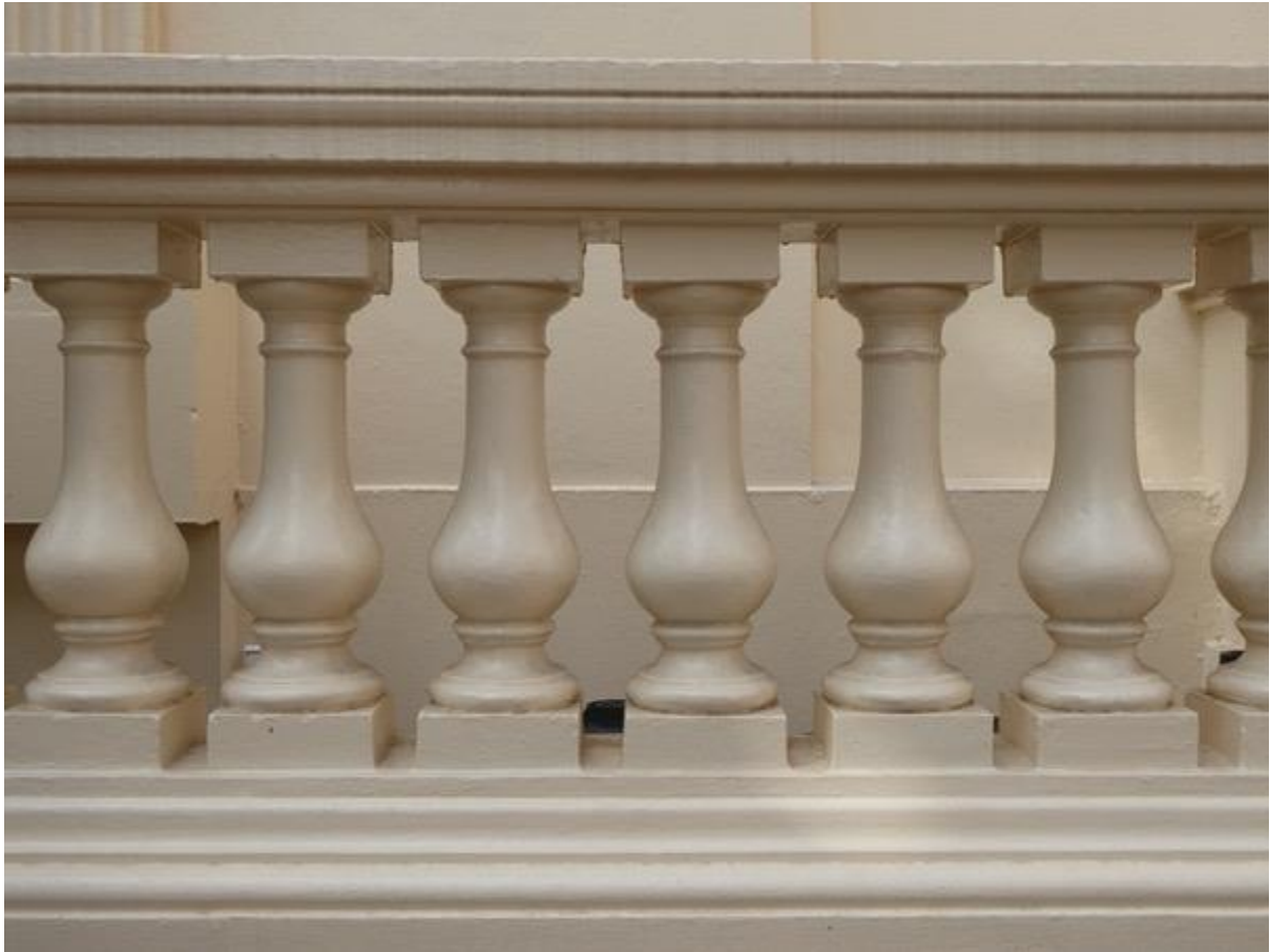
14. Proposed smooth painted finish to balustrade and plinth with no visible expansion joints
