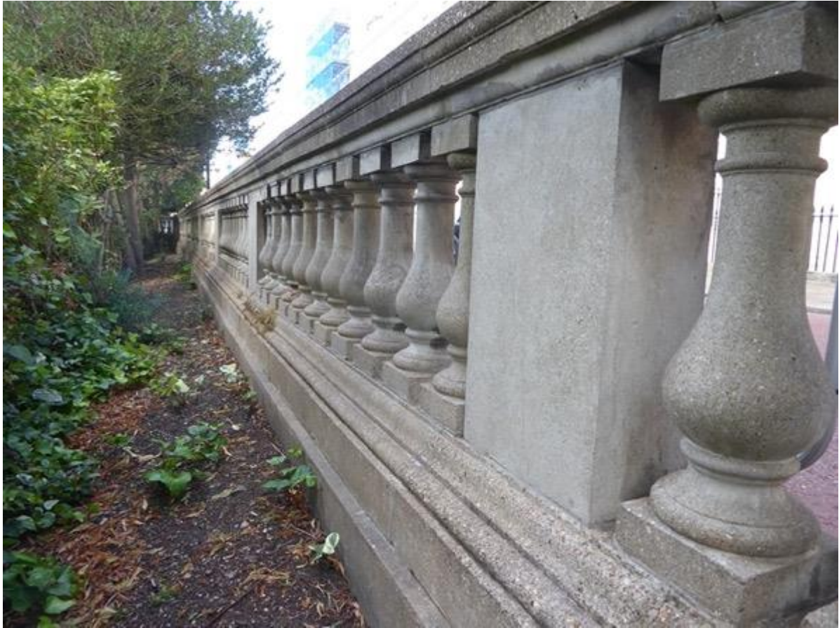
5. Chester Terrace: balustrade showing bottle balusters and plinth moulding
