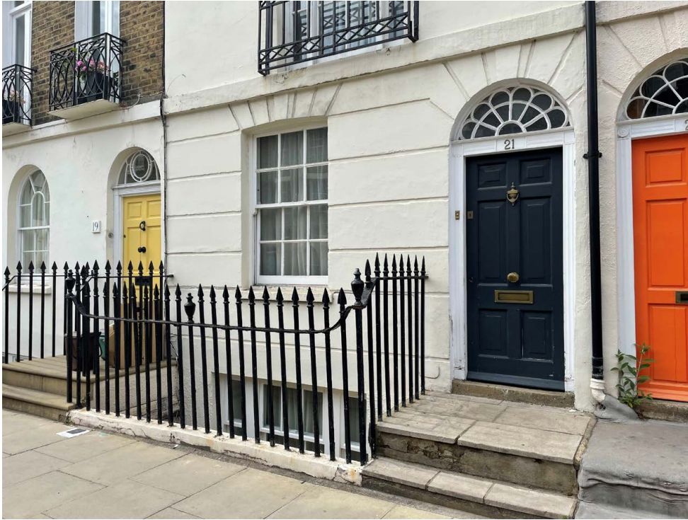
Fig. 12: Original cast iron railings to the front basement area
