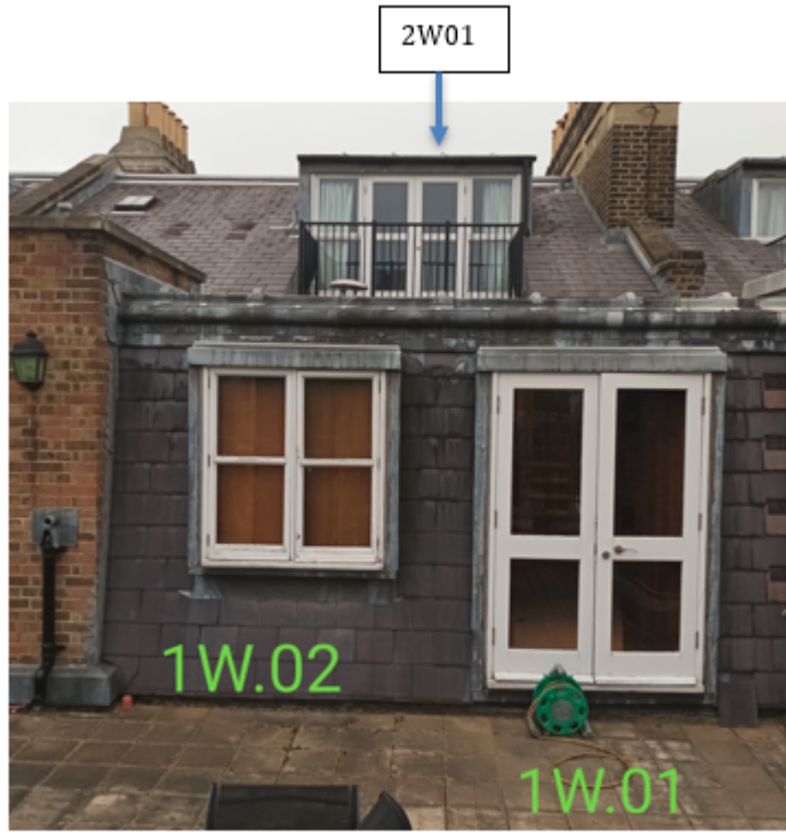
Photo 3: Windows on rear elevation (fourth and fifth floor) where secondary glazing is proposed
