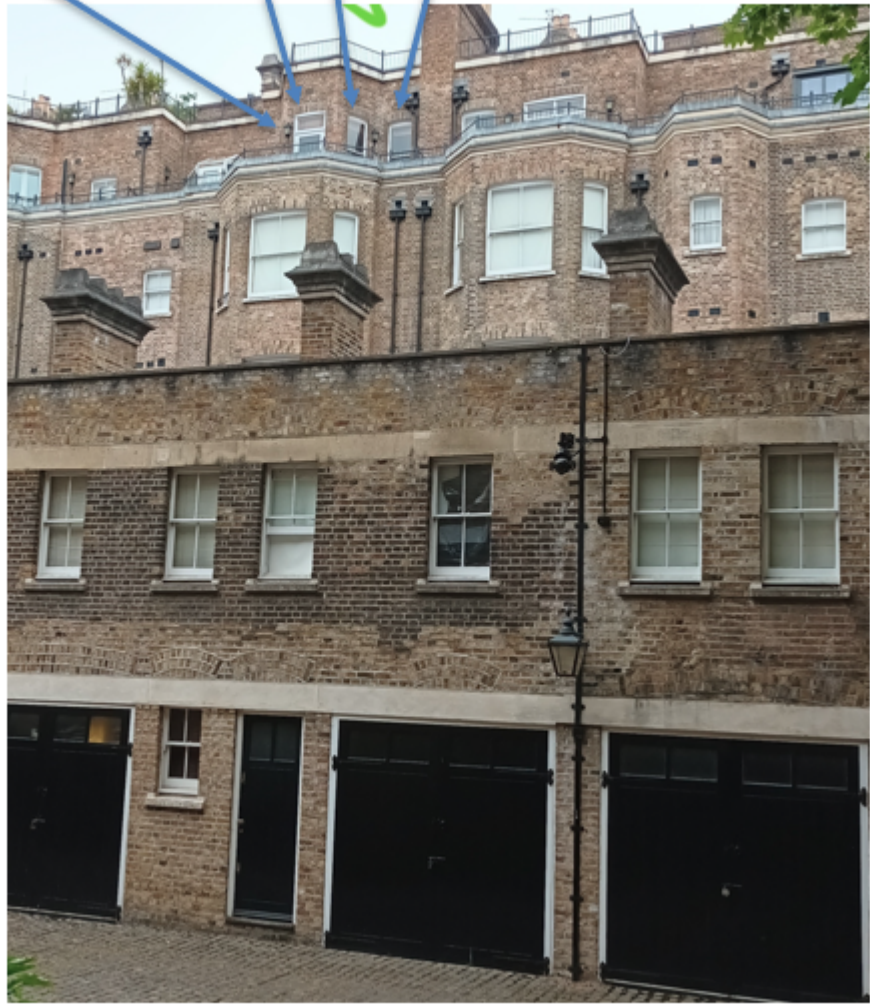
Photo 2: Windows on rear elevation (third floor) where secondary glazing is proposed
