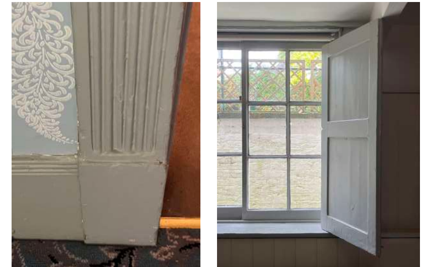
Keats House: Plinth block moulding and timber shutter in the kitchen
