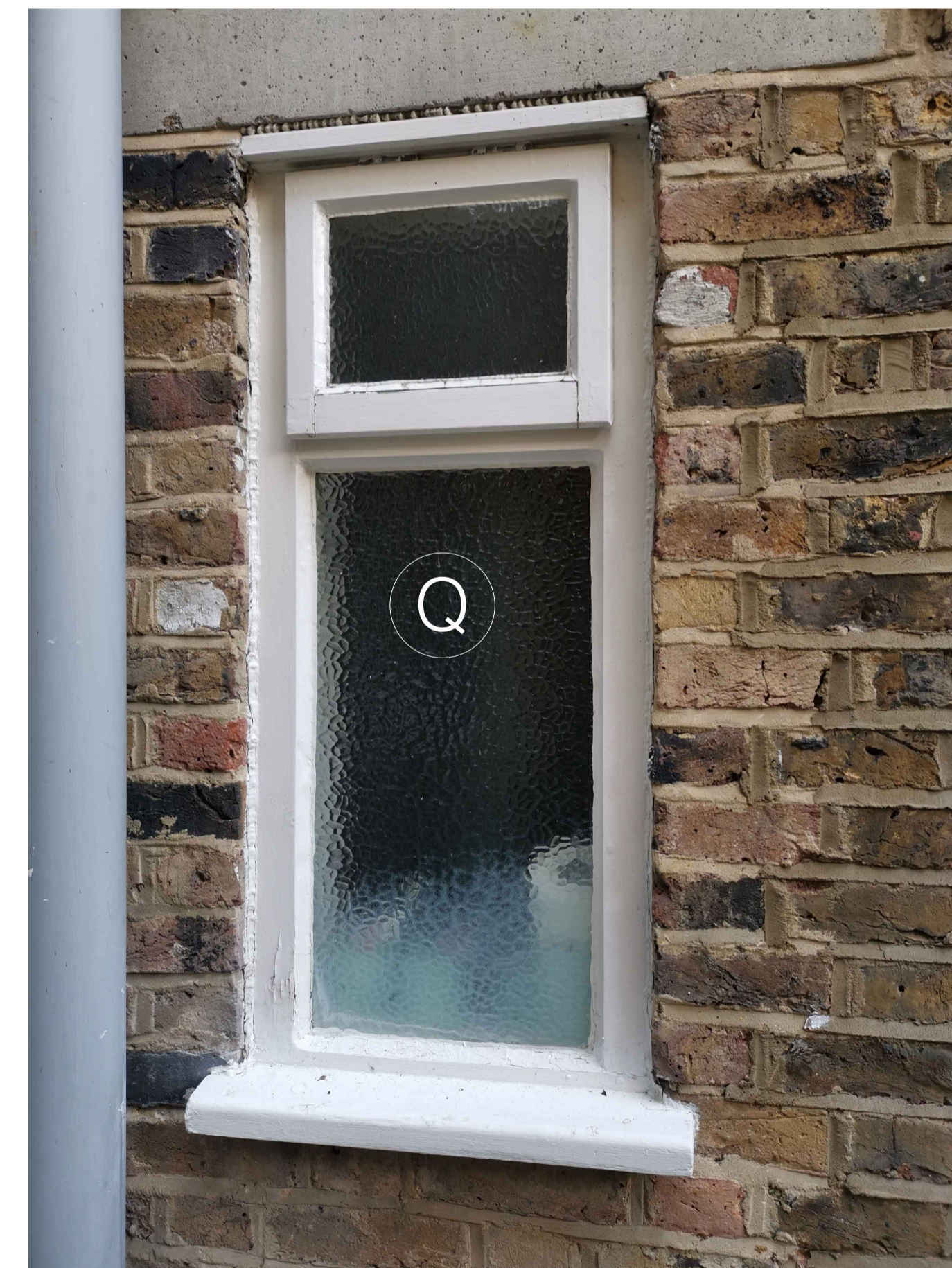
4 59 MESSINA AVENUE - EXISTING FLANK/SIDE ELEVATION PHOTOGRAPH - NOT TO SCALE
