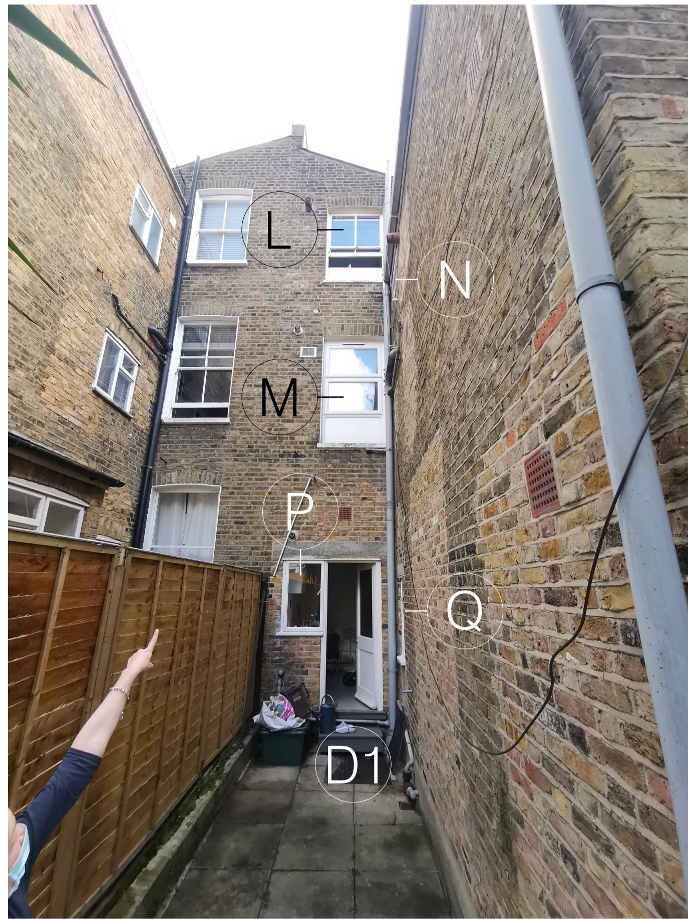
1 59 MESSINA AVENUE - EXISTING REAR ELEVATION PHOTOGRAPH - NOT TO SCALE
