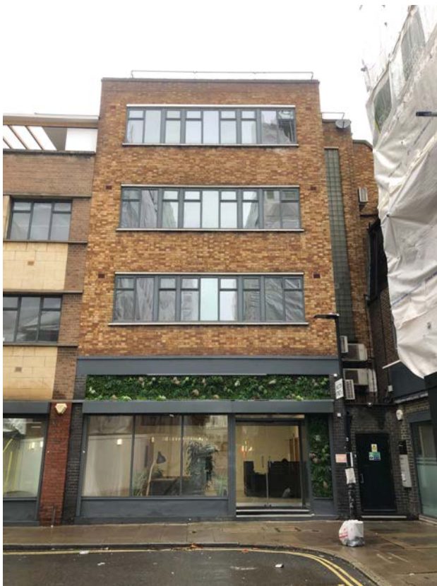
Photograph of existing 71 Shelton Street front Elevation
