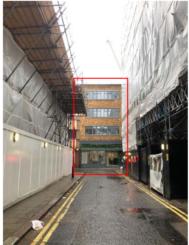
View from South East Arne Street Approach
