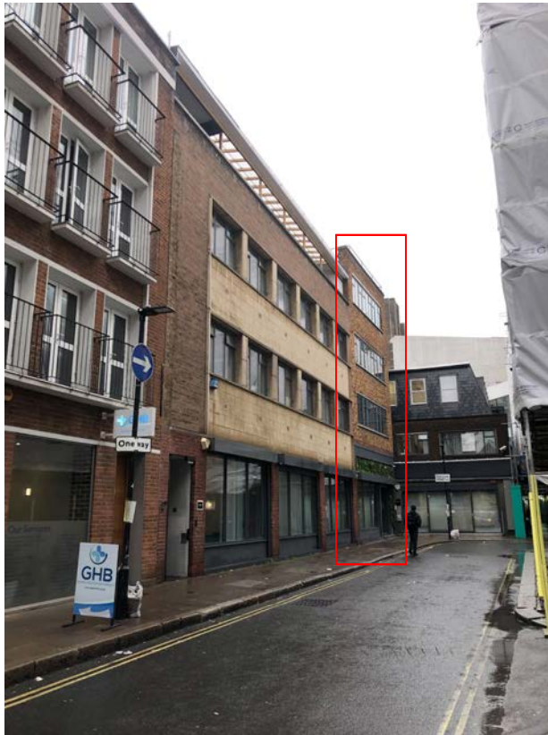
View from South West Shelton Street Approach
