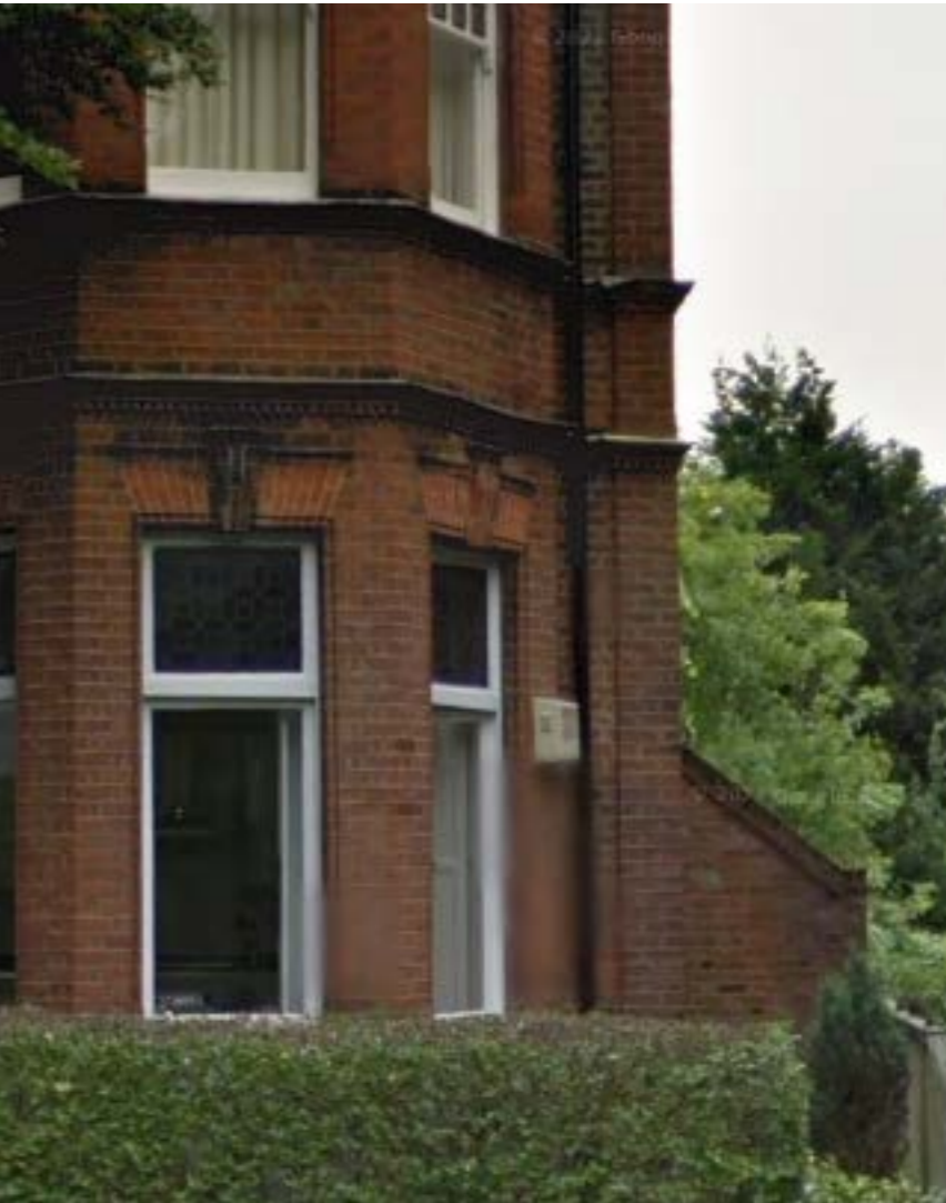
Side extension, view from the front elevation
