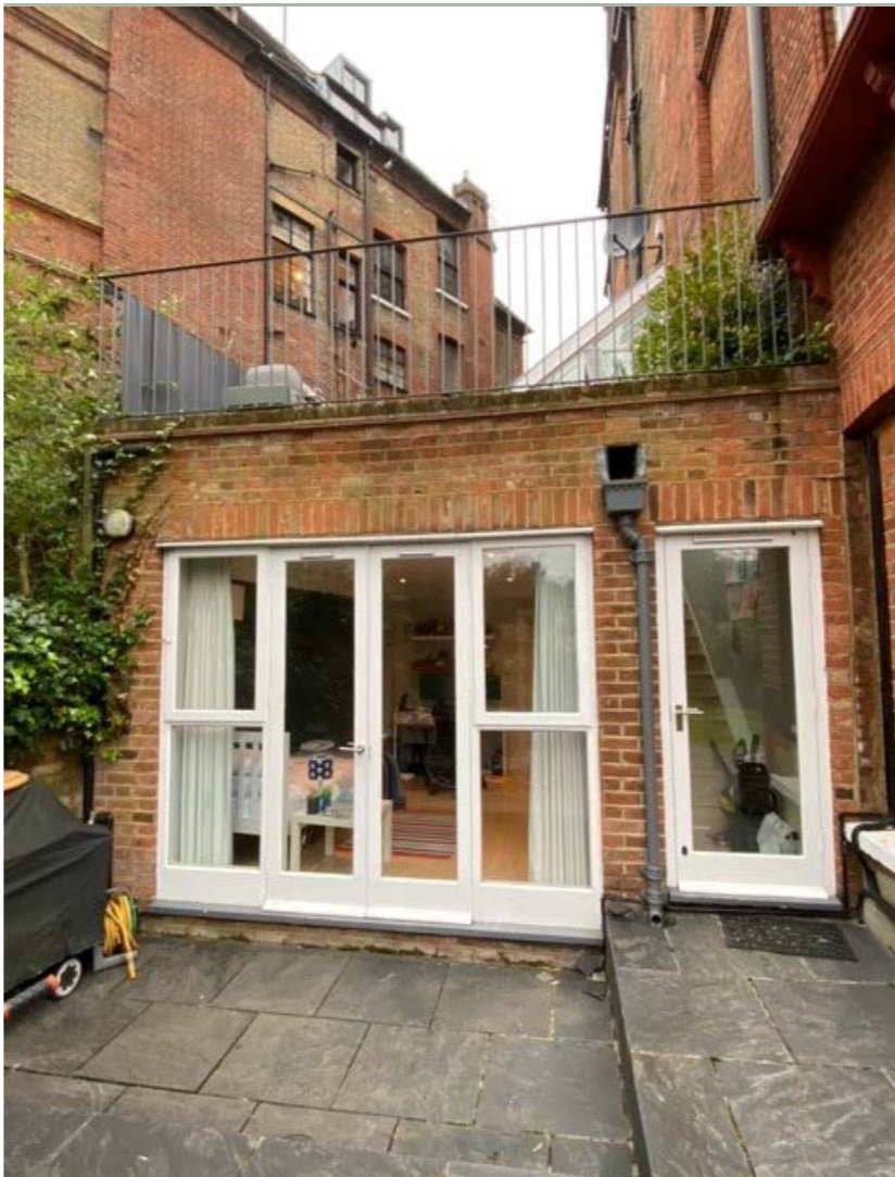
Existing LGF rear extension
