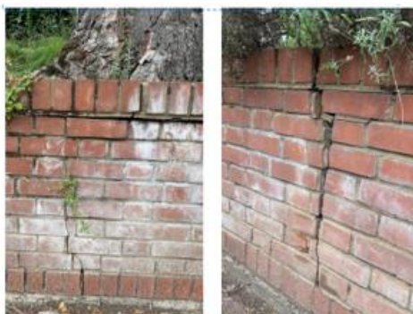
6. Cracks to retaining wall at base of Sycamore tree. [July 2021]
