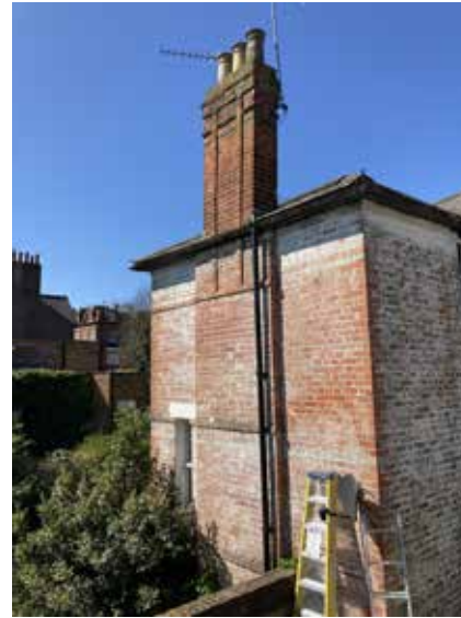
No.38 from Rear Outrigger roof
