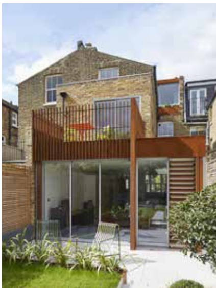
Use of Corten steel and glass in London extensions
