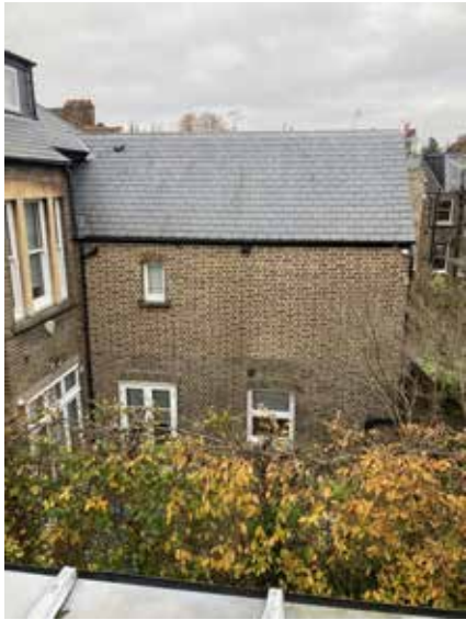
No.34 from Rear Outrigger roof
