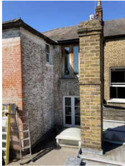
No.38 from Rear Outrigger roof
