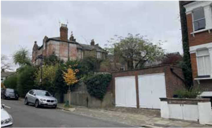
Rear of No.s 30/32 Willoughby Road seen from Carlingford Road
