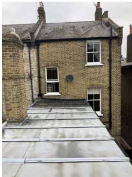
Rear elevation from rear outrigger roof
