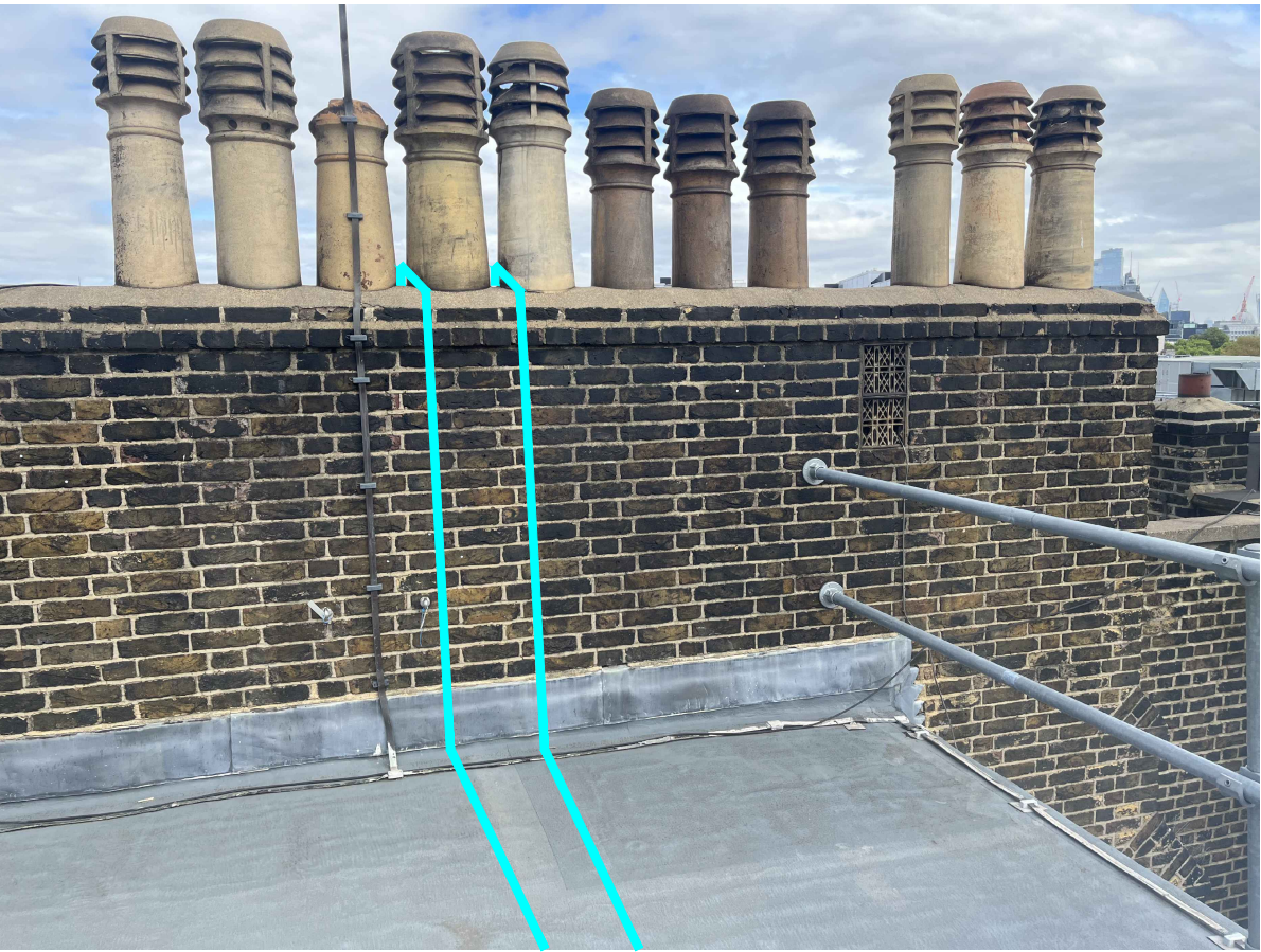
PIPE RUN OVER CHIMNEY
