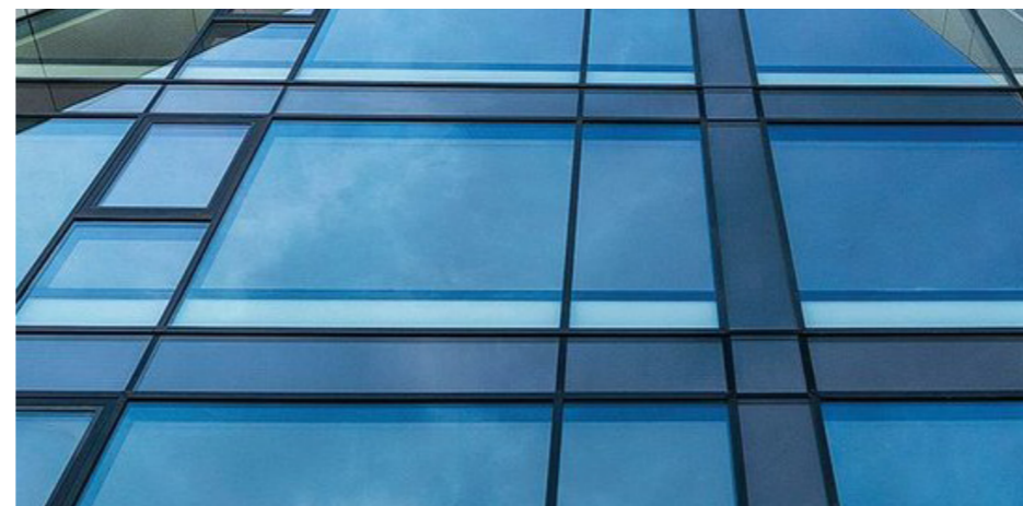
Example of dark grey curtain walling with clear and spandrel panels
