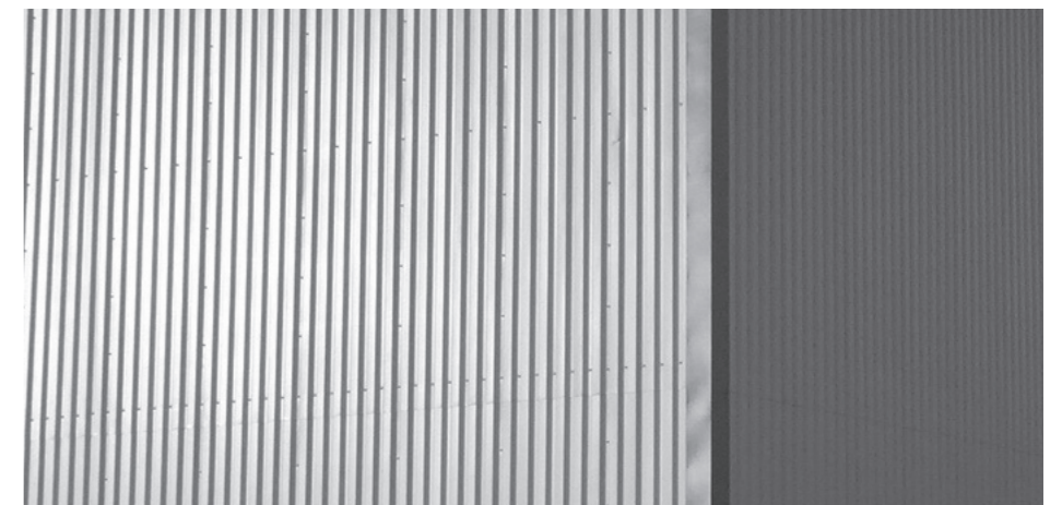
Example of grey profiled metal cladding
