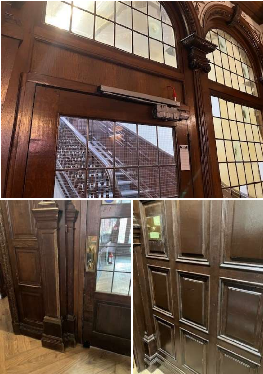
Figure 22 – Door 3. Top image showing the existing mechanism, which will be replaced by a new unit, and require a backing plate to address the shallow recess above the door. Proposed locations for the internal command points. The lower left image is taken from the entrance hall looking into the stair hall. The lower right image is of the stair hall panelling which appears to be made of poorer quality material and a lower level of craftsmanship. As noted elsewhere, the command points are wireless and their placement is reversible.
