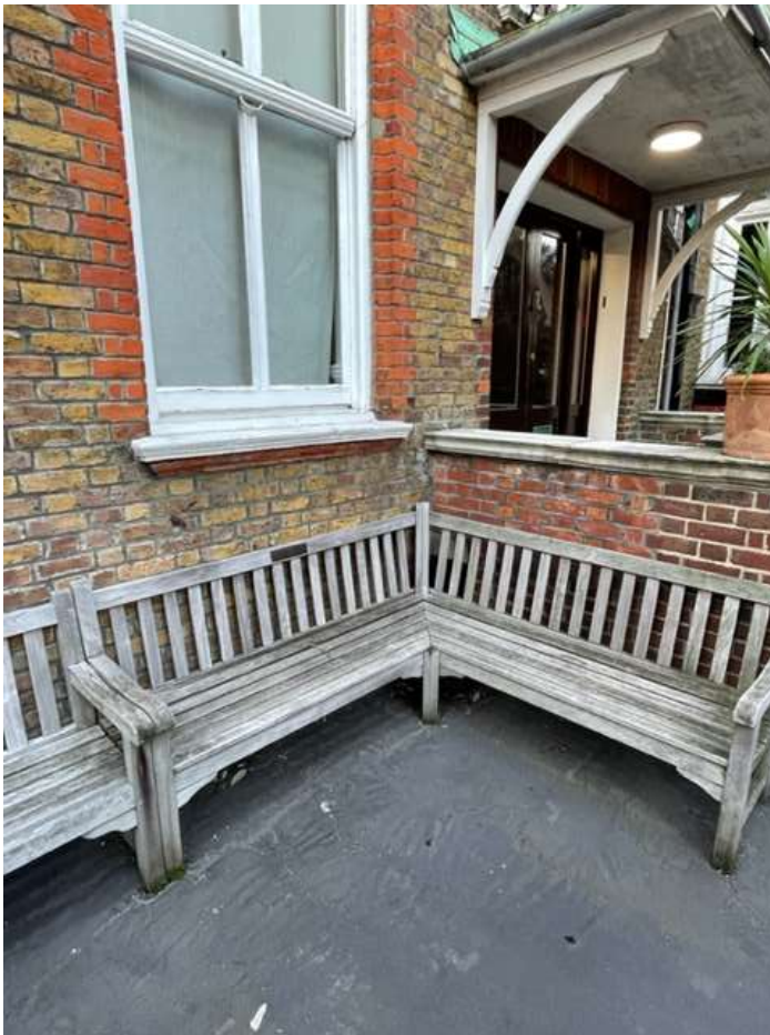
Figure 10 – Proposed location of the external lift and low wall requiring partial removal. Note the mismatched brickwork across the face of the low wall, suggesting it has been rebuilt in recent years.
