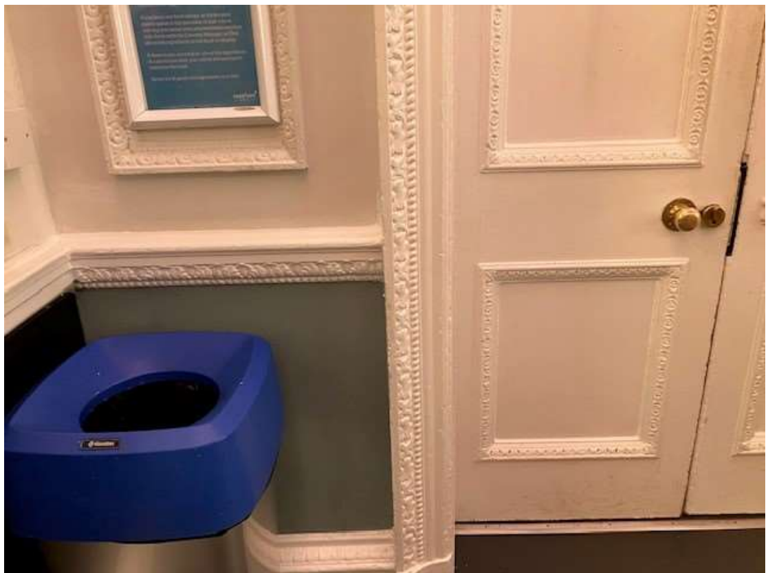
Figure 23– Door 4. Mechanisms will be placed on the entrance hall side of the opening, avoiding direct or indirect impacts to the rich decoration of the entablature on the common room side. The call point for this side of the door will be placed below the dado rail to minimise any adverse impacts arising through introducing a visually discordant element into an area of particular aesthetic value.
