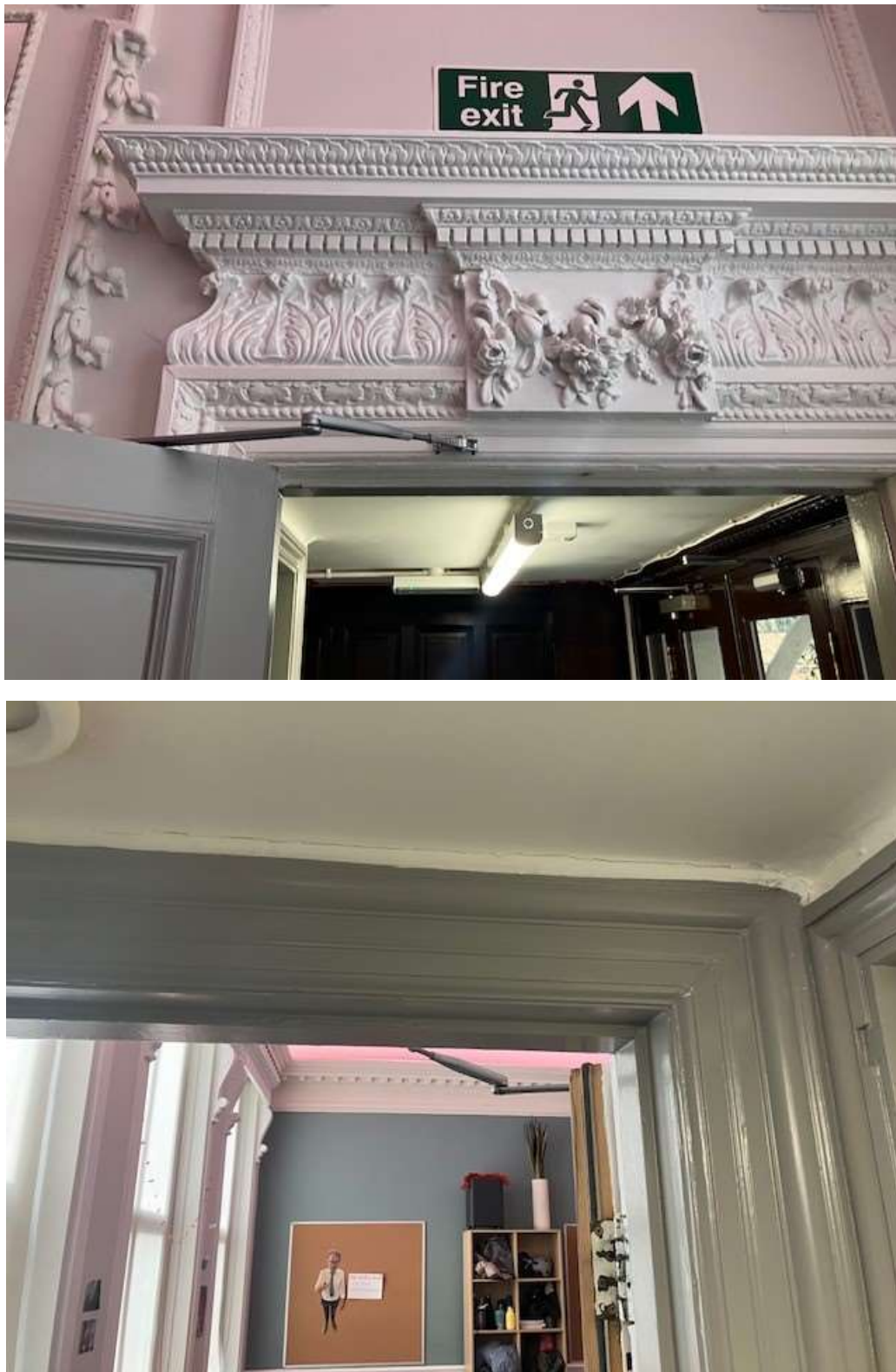
Figure 20 – Door 2. The highly decorative door surround on the common room side of door 2 (top image), through its aesthetic value and size, meant any automation mechanisms in this location would be entirely problematic. The proposal as part of this application is for the mechanism to be located on the other side of the wall, while keeping the existing opening direction. In order for the unit to operate properly, a piece of architrave above the door will need to be removed so the opening mechanism can sit flush against the wall. Despite many options being tested, a less invasive solution has not been identified.
