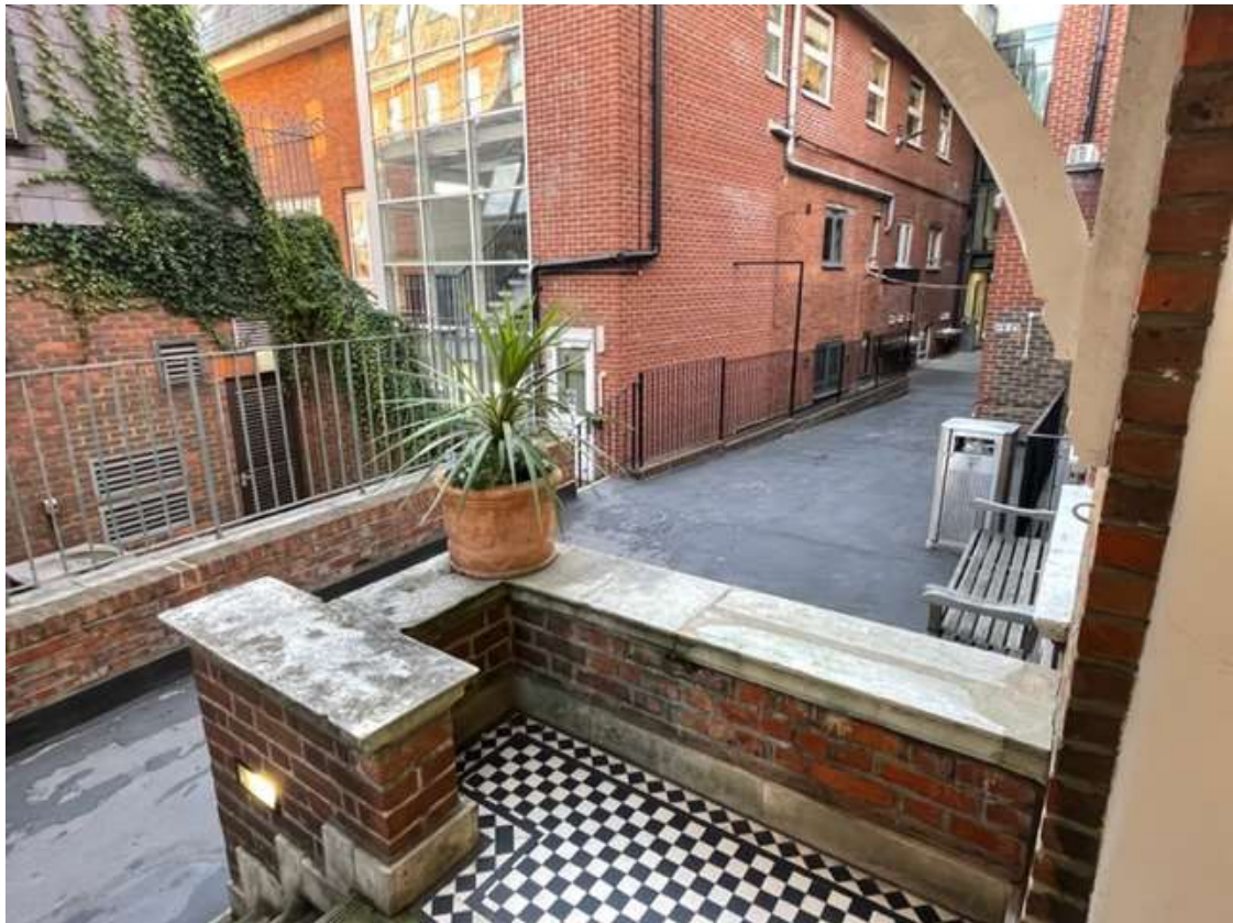
Figure 11 – Proposed location of the external lift and low wall requiring partial removal. Again, note the poor brickwork and differing colour of the bricks in the section proposed for removal.
