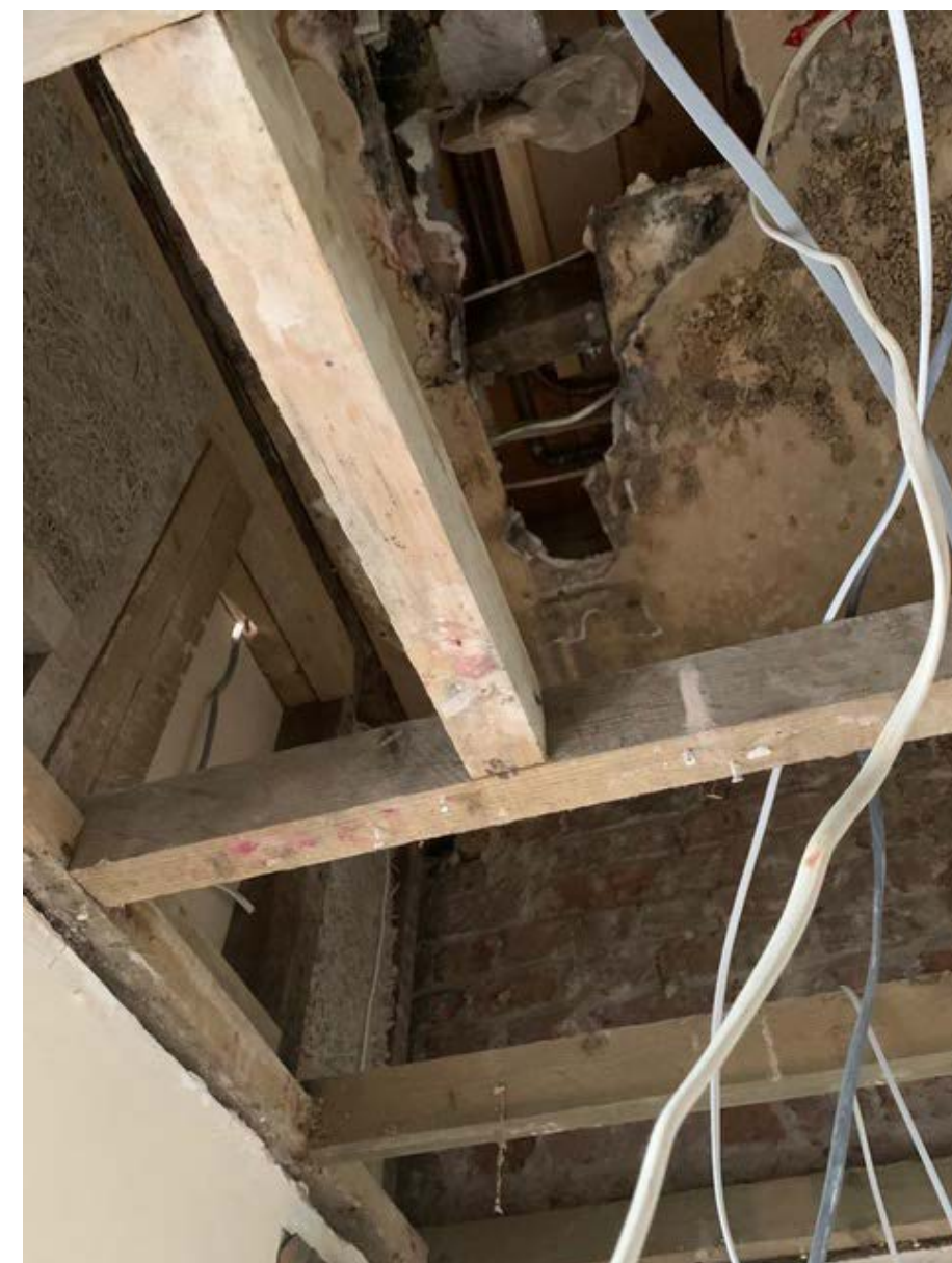
Uncovering of ceiling plasterboard has brought discovery of floor above with a significant hole underneath the bath in the bathroom.
