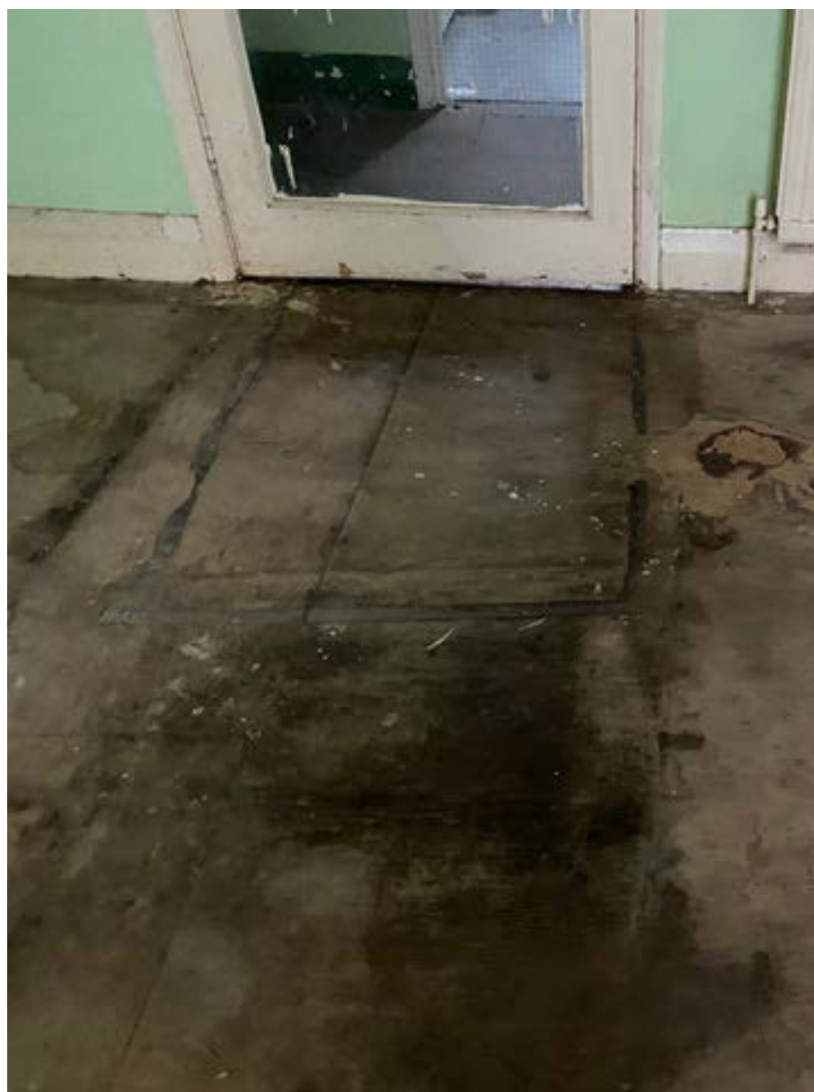
Floor showing signs of water ingress.
