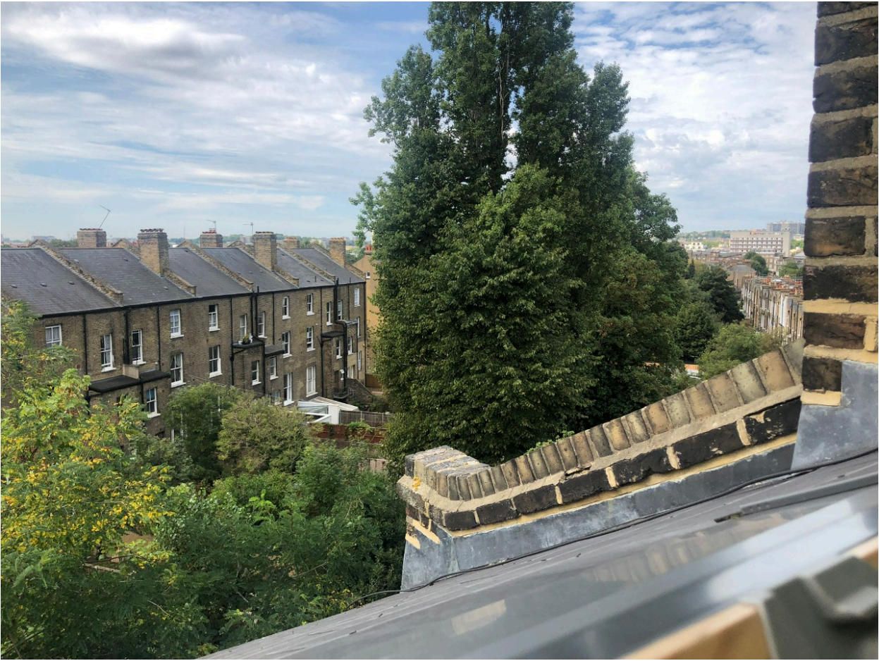
Figure 2. Views out from rear roof lights overlooking London rooftops
