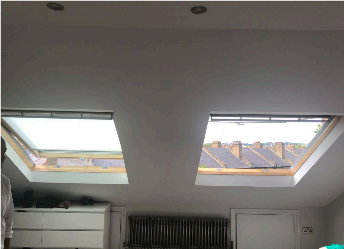
Figure 3. Views out from rear roof lights from master bedroom
