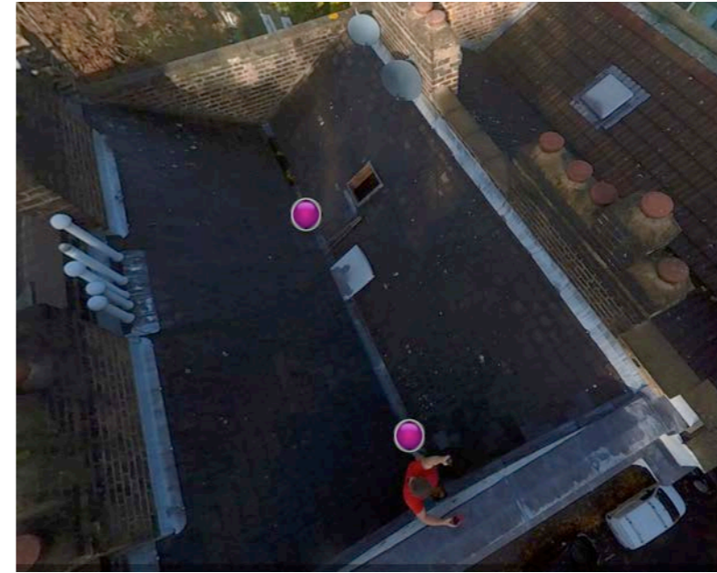
4 Aerial View of Roof
