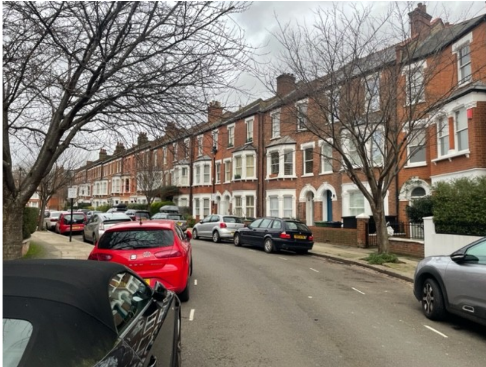
Above: View of the constructed cycle shed (centre right) looking north on Mackeson Road
