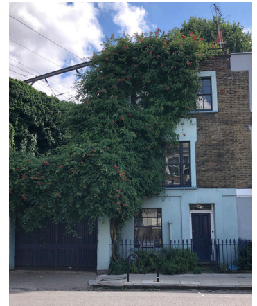
Existing street elevation 32 Hartland Road
