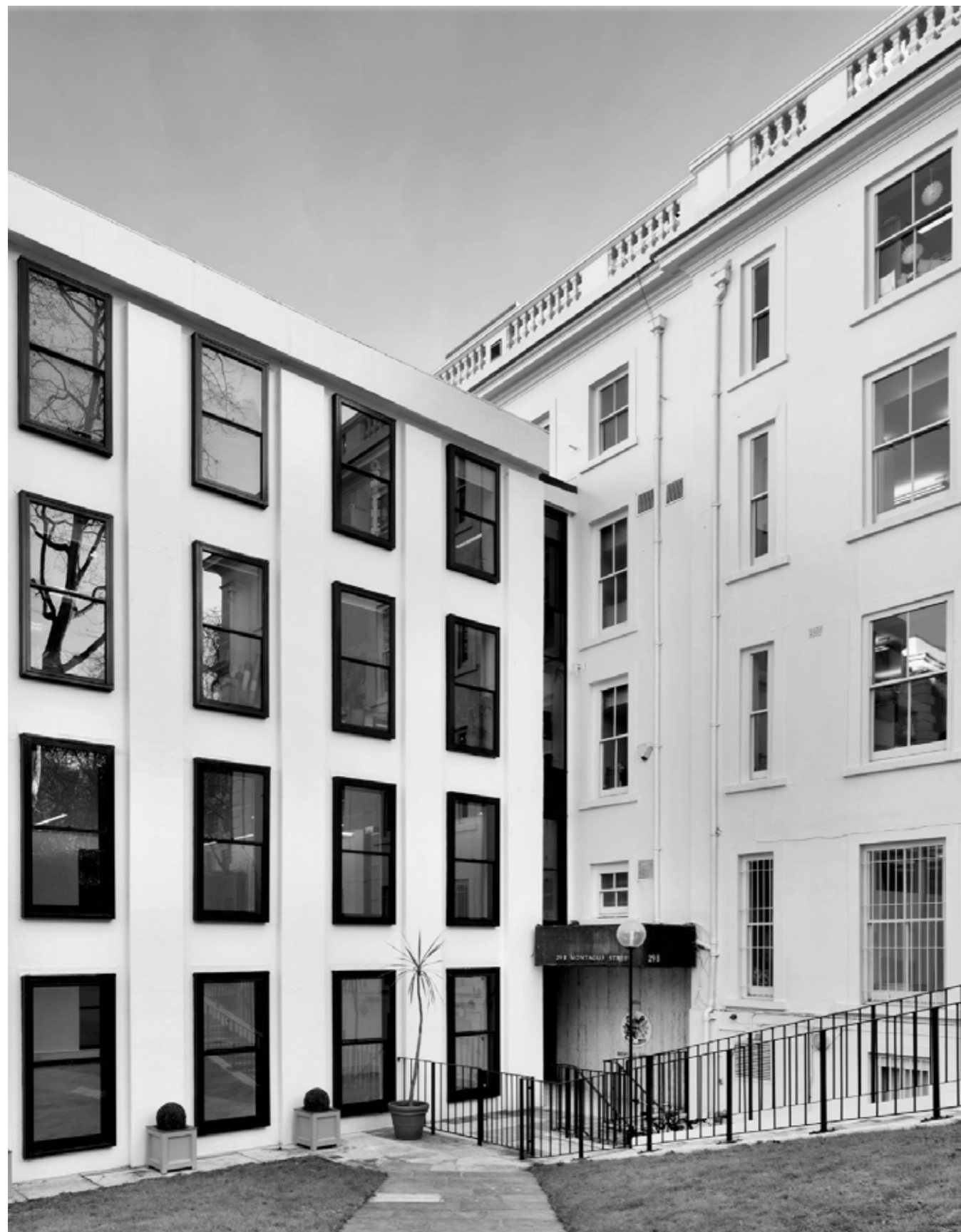
Left: View from the enclosed front garden of 29A-B, looking towards the entrance of 29B at lower ground.
