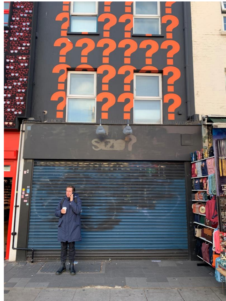
261 Camden High Street: Existing Shopfront with the shutters in closed position.
