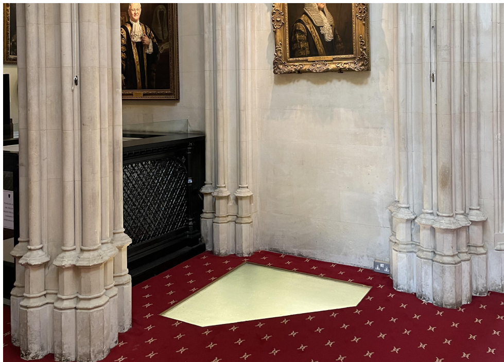
4. Floor light next to existing lift
