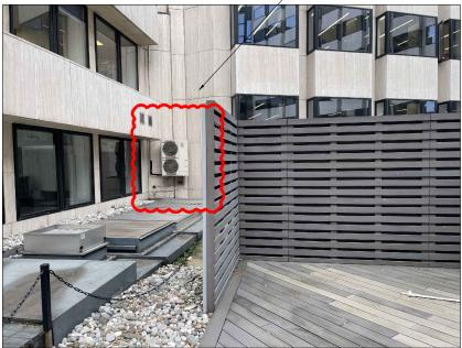
efrigerant shall rise up the building Contractor to agree penetration location, fire seal, facade finish and waterproofing detail with architect prior to carrying out any works
