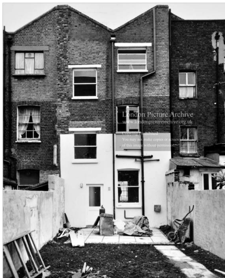
Figure 18: Rear elevation of No. 123 (No. 125 visible to the left) photographed in 1975 following the removal of the rear outrigger and party wall projecting end stack. The shadow of the chimney stack remains visible to the partition with No. 125 (note rough brickwork to former flue lining). © London Picture Archive Collage Ref. 106214.
