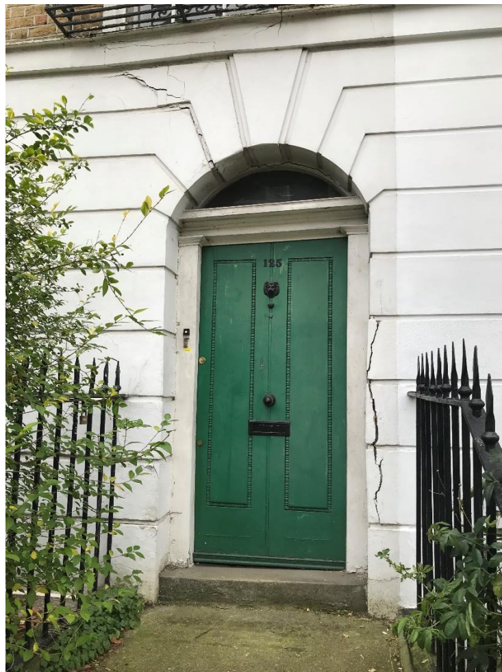
Figure 5: Entrance door to No. 125 showing evidence of settlement to the front masonry wall and cracking / movement to the stucco finishes.
