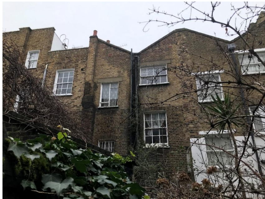
Figure 4: View of the rear elevation. No. 125 corresponds to the central two bays beneath the V-shaped parapet. Note the remodelled second floor / mezzanine windows with concrete lintels.
