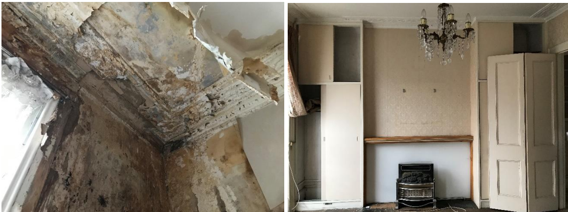
Figure 21: The most ornate plasterwork cornicing is at first floor level and is similar to the front and rear rooms. It has been heavily damaged by water ingress in the kitchen (left) or obscured by fitted cupboards in the bed-living room (right).
