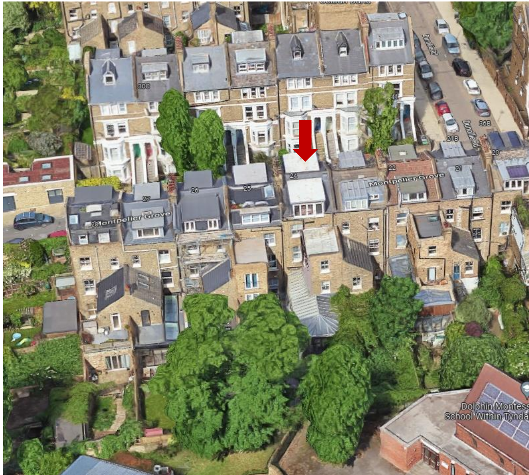
Figure 3. Close-up aerial view looking east (site marked with a red arrow) © Google
