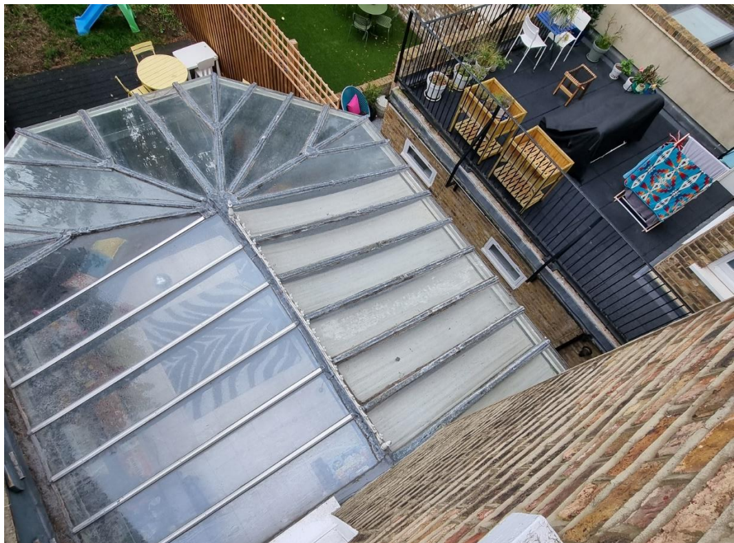
Figure 5. View of the existing poor quality ground floor extension from above. Note the roof terrace to no. 25's flat roof (top right-hand side) © SEB + FIN Architects
