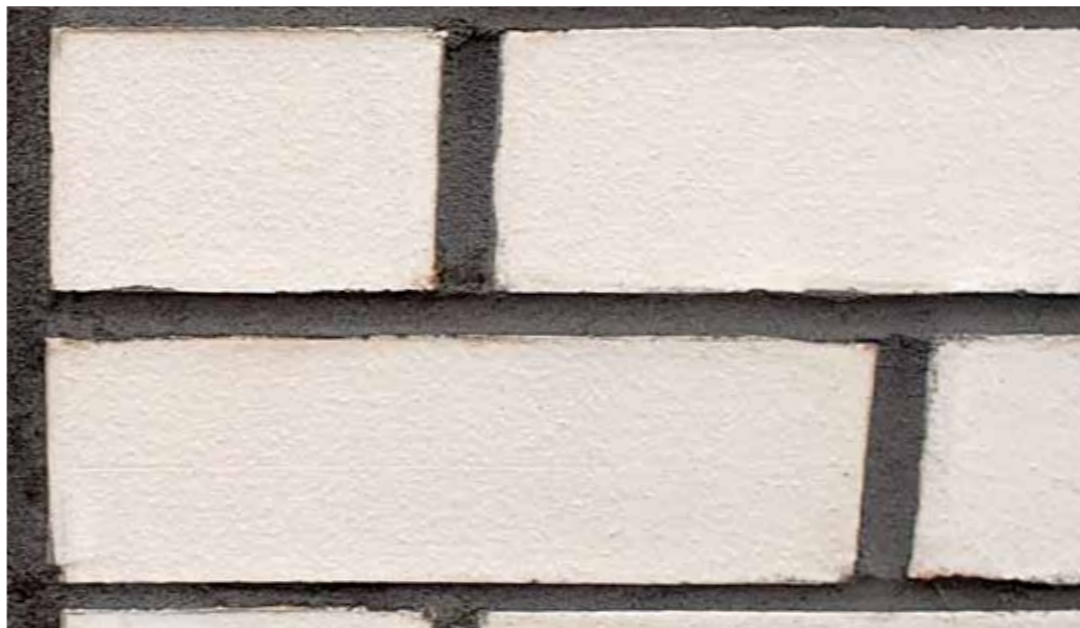
Detail of white smooth facing brickwork
