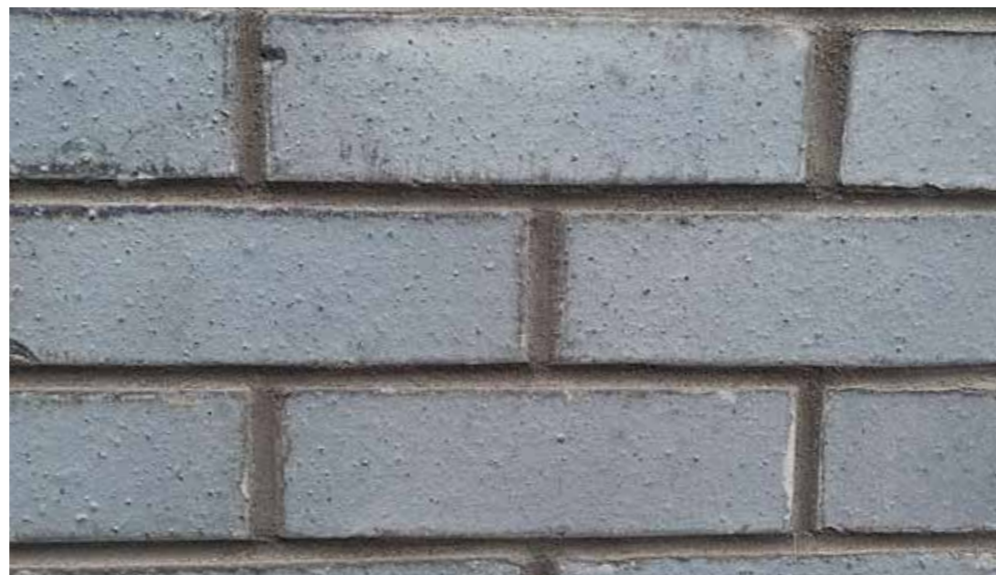
Sample panel 03 - illustrating White smooth facing brick. Dark coloured brick trim and panels are Black smooth brick, see sample panel 04 for manufacture reference.
