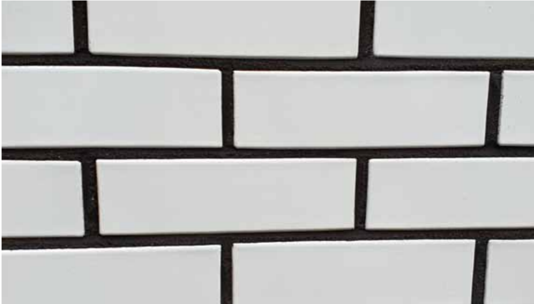
Detail of white glazed facing brickwork
