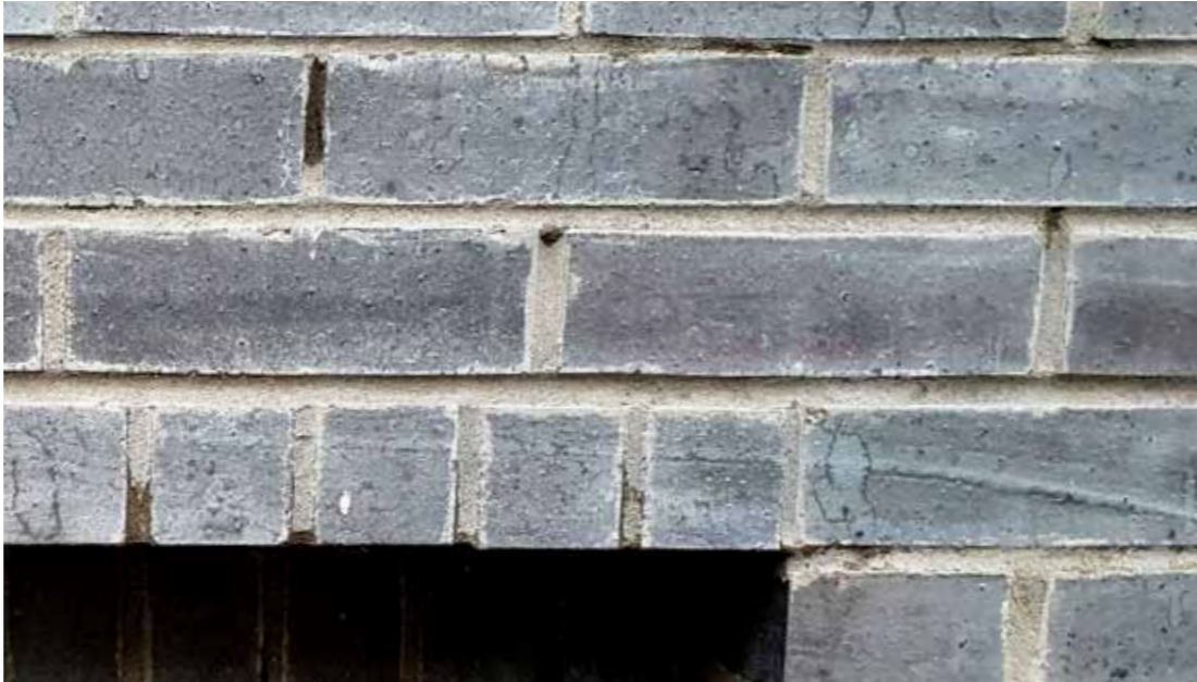
Detail of white smooth facing brickwork
