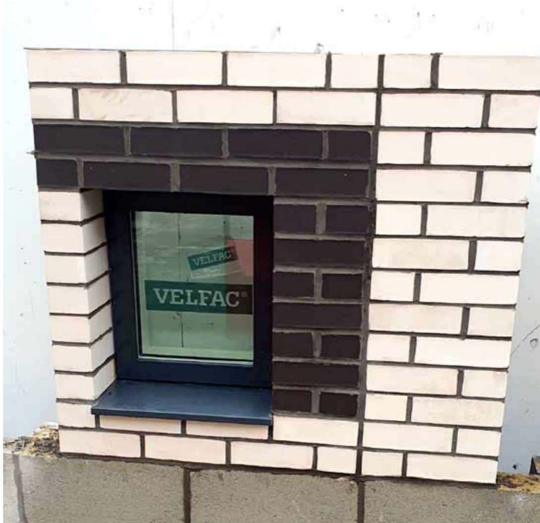
Sample panel 02 - illustrating White smooth facing brick. Dark coloured brick trim and panels are Black smooth brick, see sample panel 04 for brick type and manufacturer reference.
