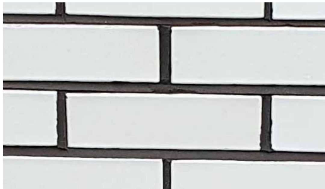
Detail of white glazed facing brickwork
