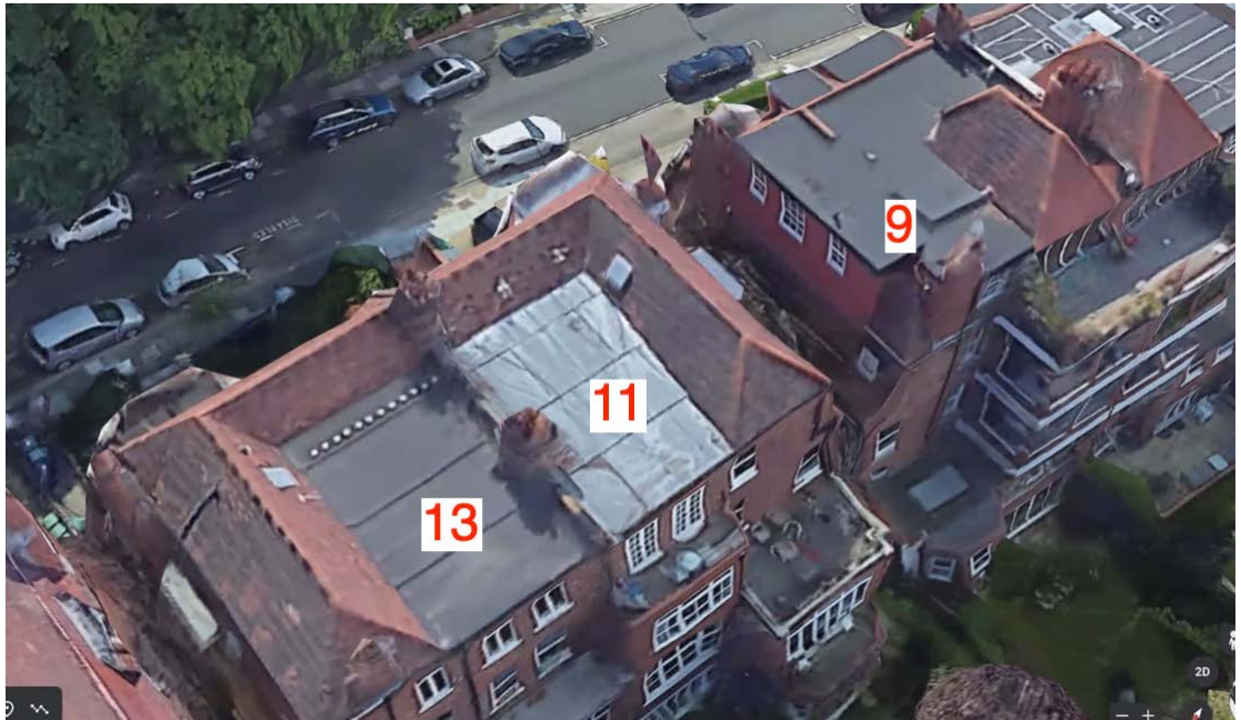
Fig 4: Aerial view of 11 Langland Gardens showing the existing flat roof
