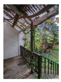
The rear of the property is fairly simple in design with three sash windows set within a red brick façade. Again, the slate roof has two rooflights. At ground floor level is a timber veranda structure with corrugated plastic roof, which is in poor condition and is a detracting feature of the property.
