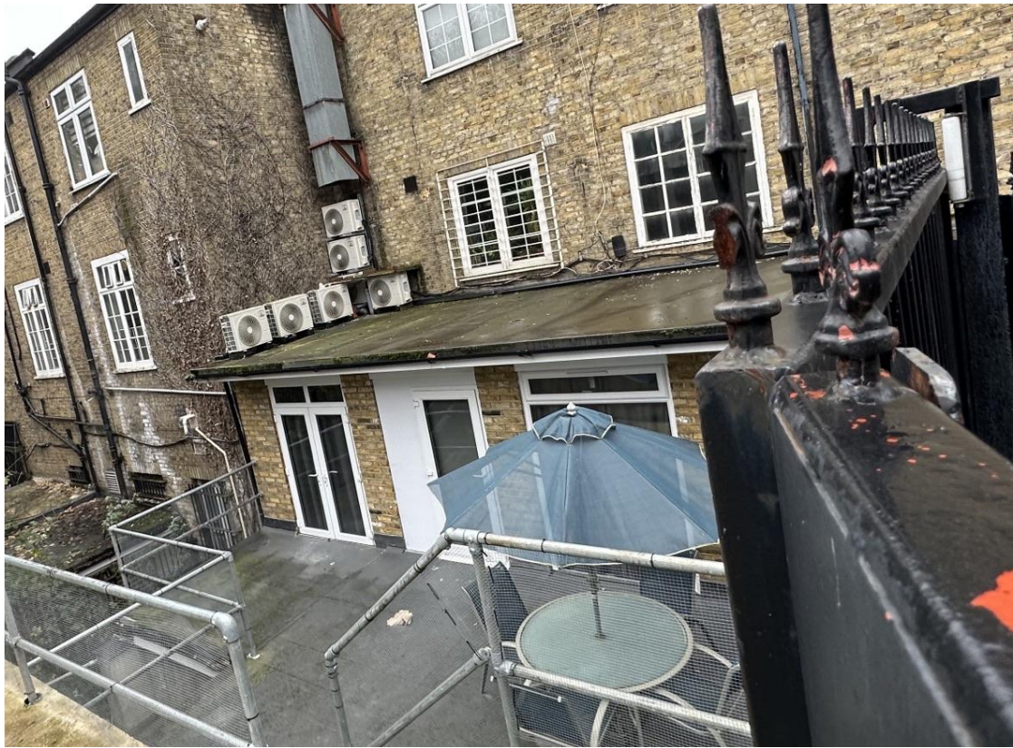
Fig 4. Showing windows and doors at the rear of the property
