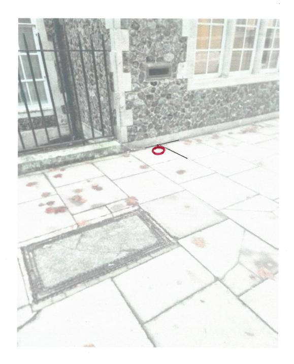
New 54mm duct to be created via core drill, beneath footpath.
