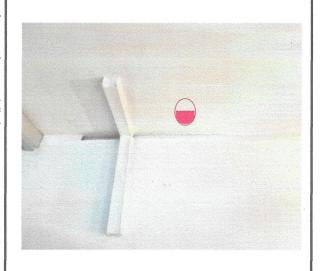
New 54mm duct to be created via core drill adjacent to existing Virgin Media orange fibre underneath mailbox within wall, which leads into void under letter box within Nuffield Entrance. Make good and tidy after core drill completed
