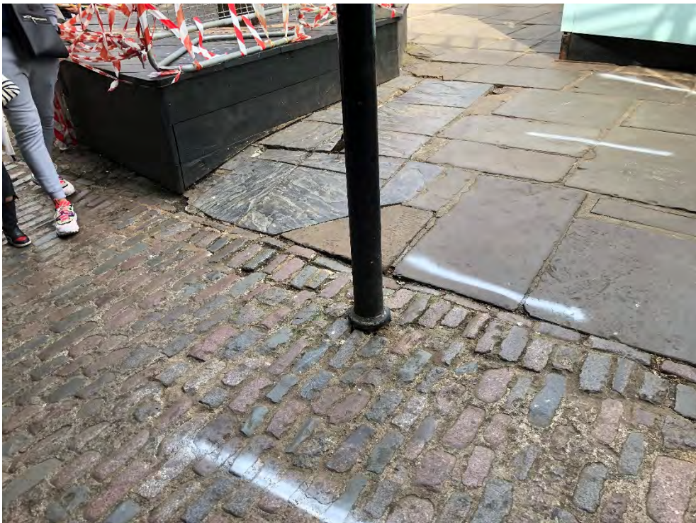
Figure 2.4: Granite setts and York Stone slabs are the common paving materials within the Site.
