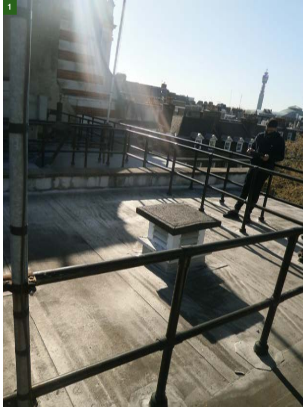
Figure 33. Existing roof over 4 BS showing ventilation cowls and showing current edge protection.
