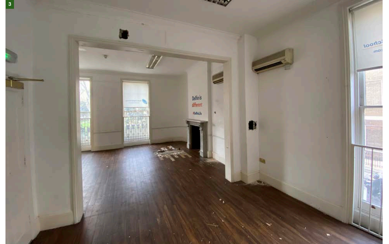
Figure 24. First floor front room within 47 BS.
