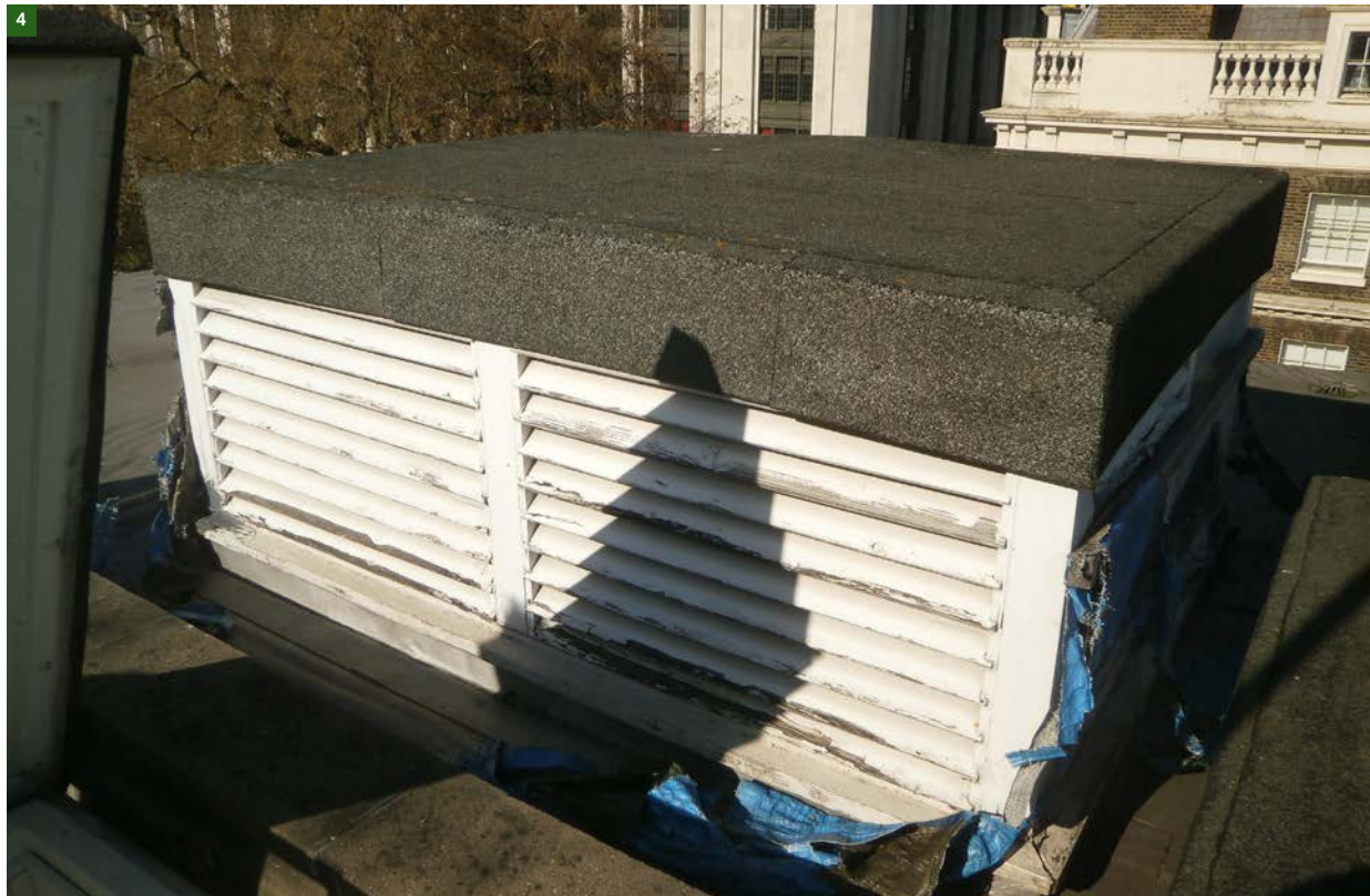
Figure 35. Existing cowl over plant room.
