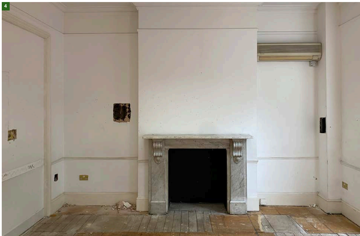
Figure 25. Existing fireplace, wall mounted FCU and in filled opening between front and back rooms in 47 BS.
