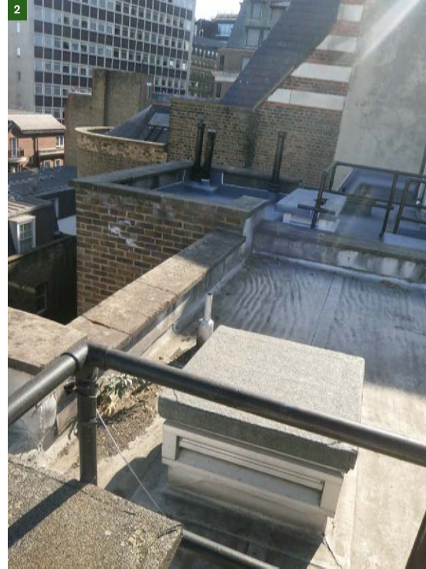
Figure 33. Existing roof over 4 BS showing ventilation cowls and showing current edge protection.
