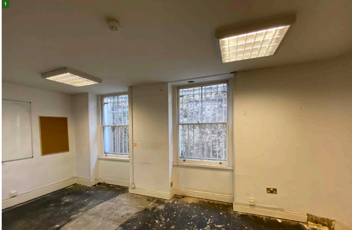
Figure 16. Lower ground front room within 47 BS.
