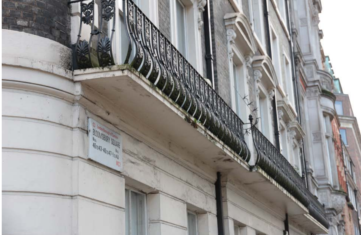
Figure 5. Existing balconies along Bloomsbury Square frontage.
