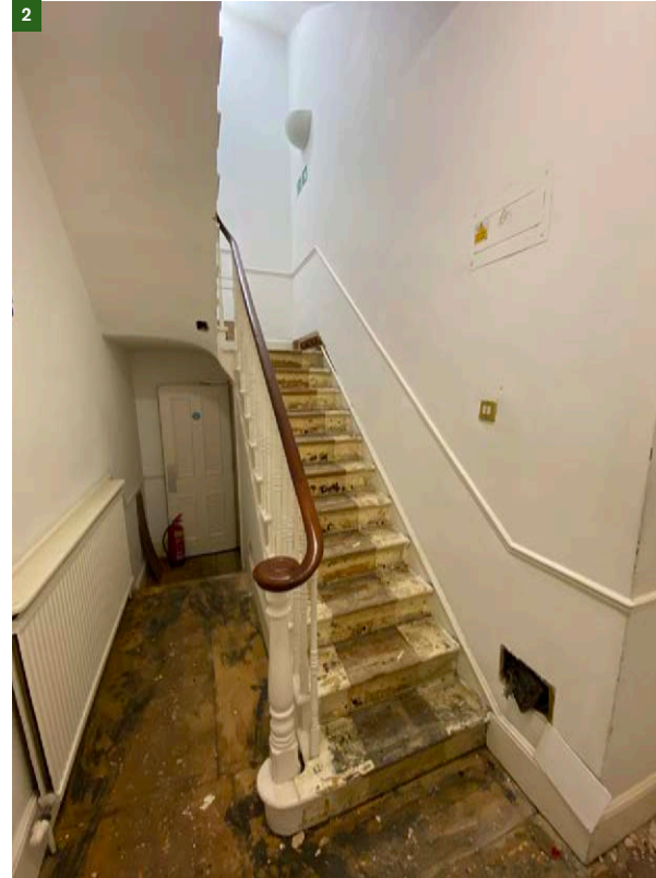
Figure 11. Existing stairs within 46 BS.
