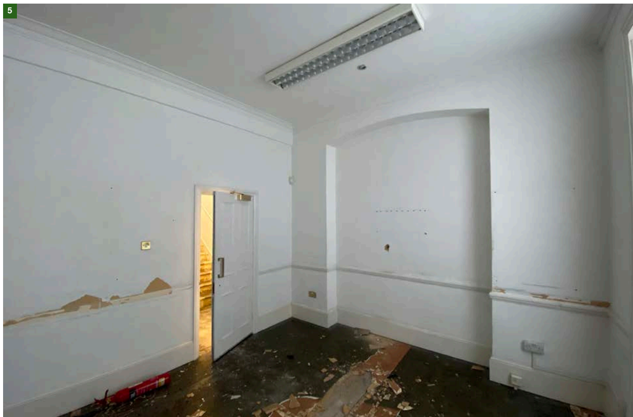
Figure 13. Existing front room within 47 BS.
