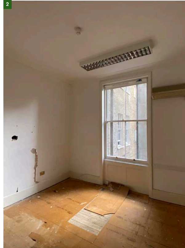
Figure 23. First floor back room within 47 BS.
