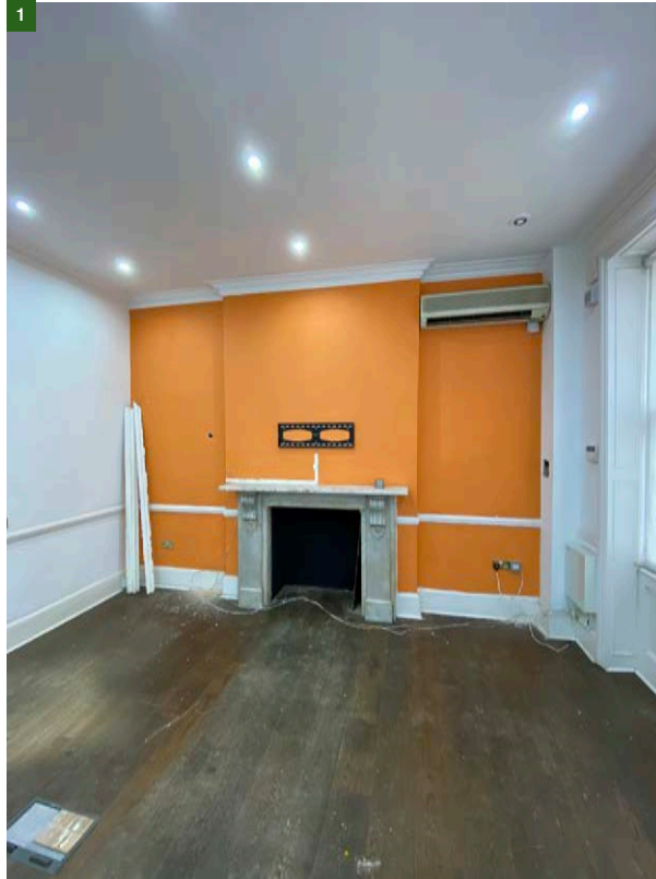
Figure 10. Existing front room within 47 BS.
