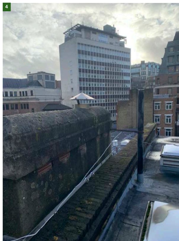
Figure 17. Existing capped chimneys.
