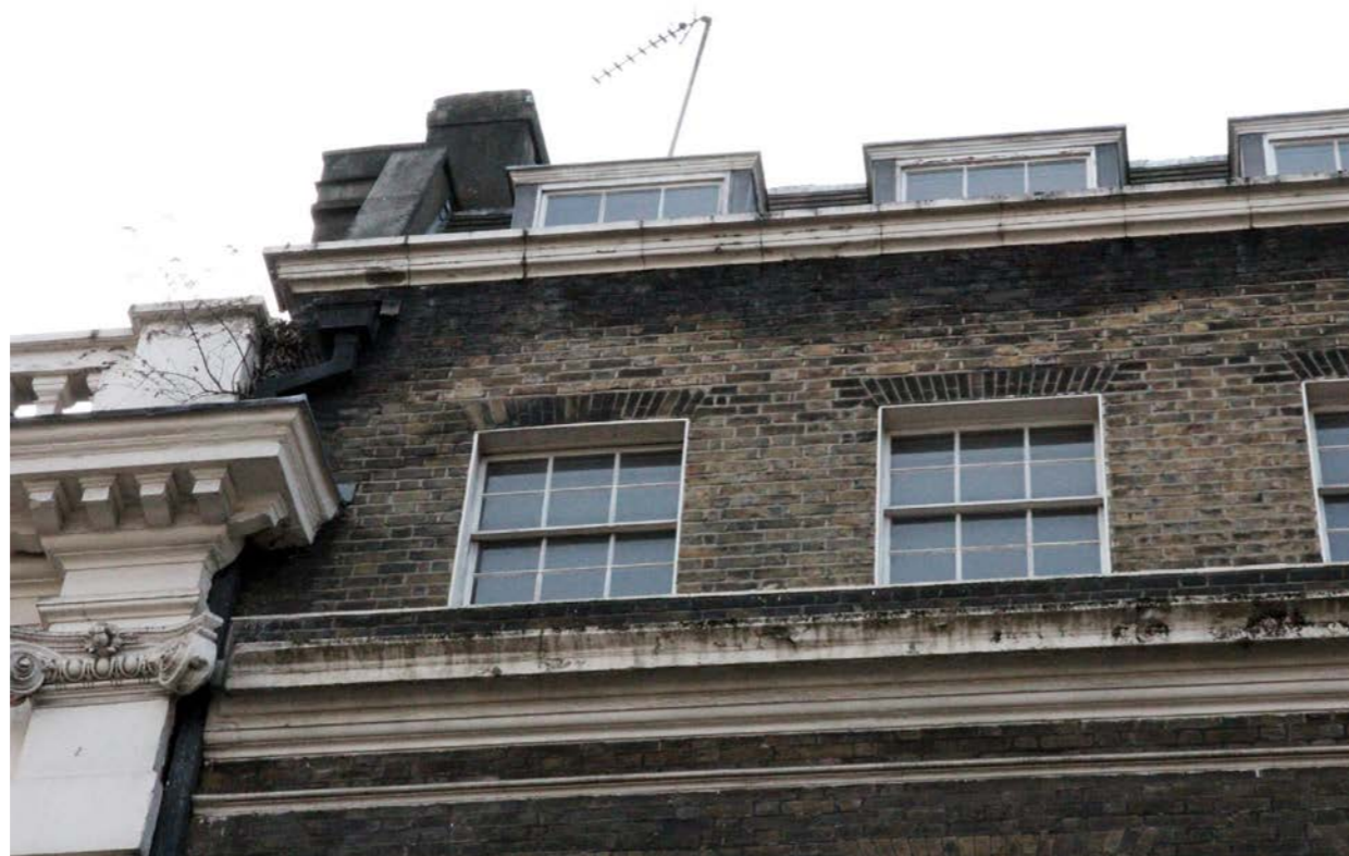
Figure 4. Existing photo of 20-21 showing façade condition.
