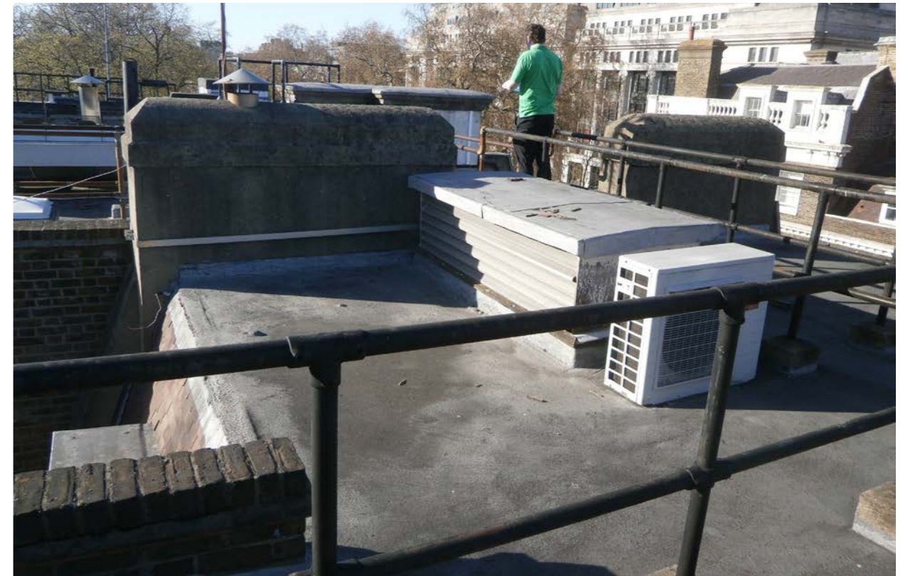
Figure 5. Roof of 21 Southampton Place looking North towards Bloomsbury Square.
