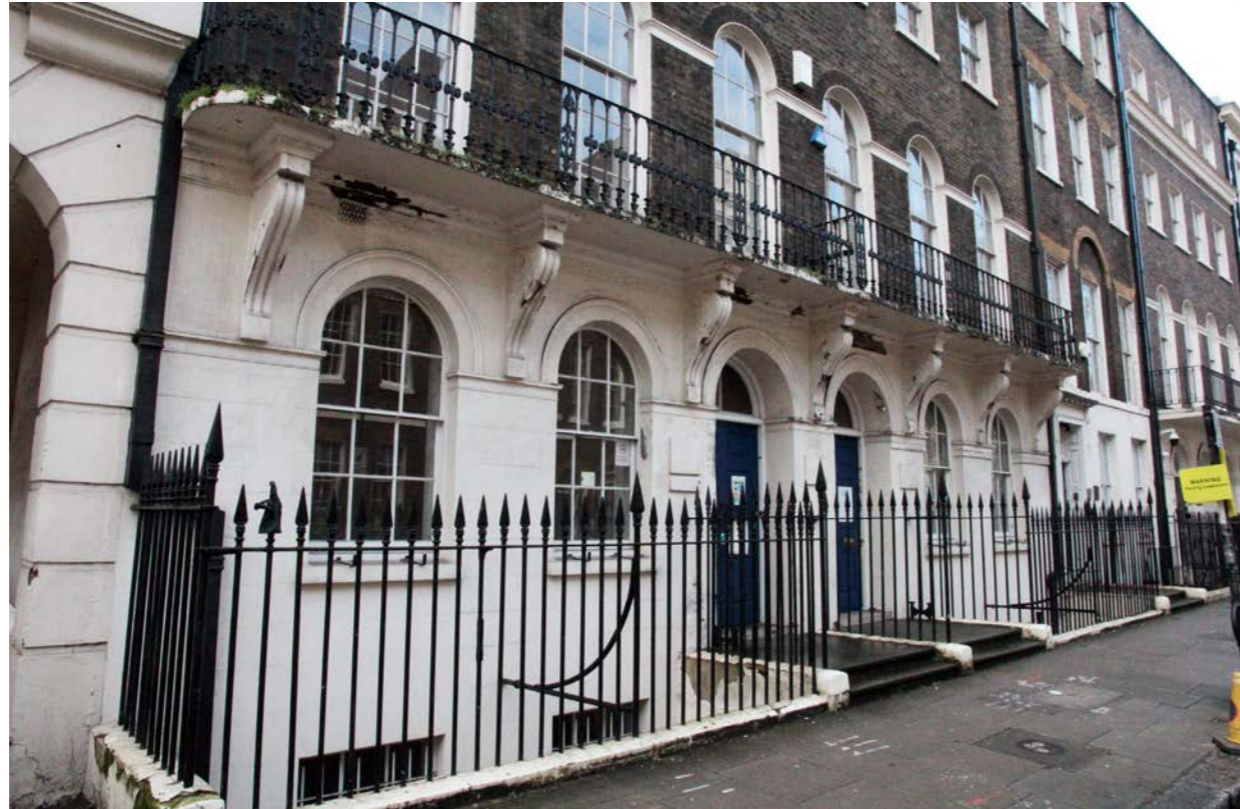
Figure 3. Existing photo of 20-21 ground floor fronting onto Southampton Place.
