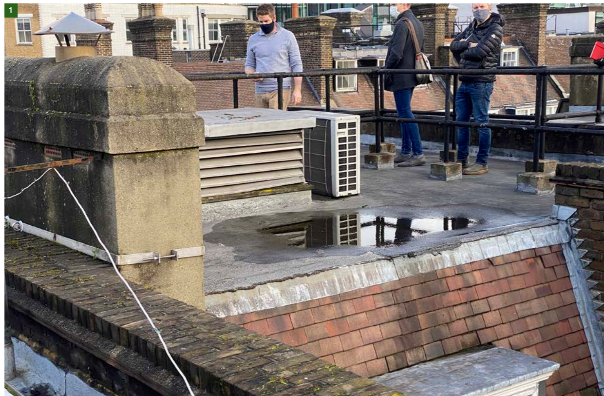
Figure 14. Existing roof on 21 SP.
