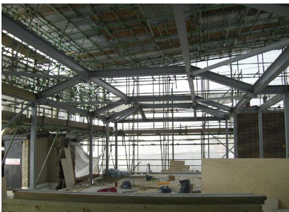
Photo 5: Primary structure erected above transfer deck on MBP's Lowndes Square penthouses
