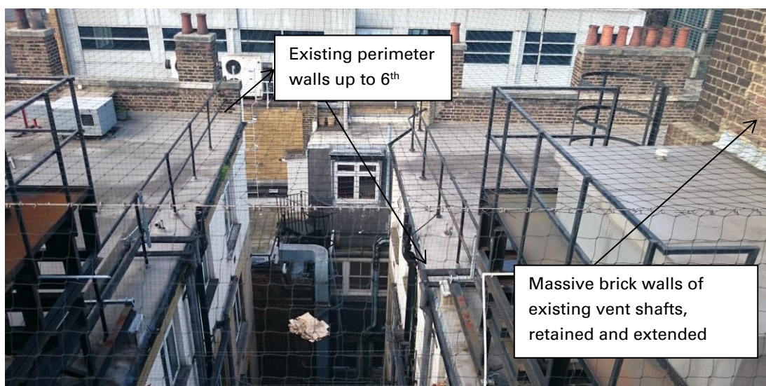
Photo 1: Existing light well and walls
