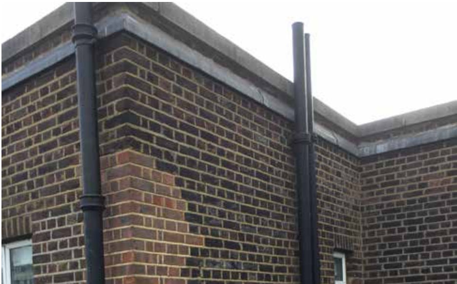
Fig 27.View of parapet detail on the existing roof level. (note lead flashing added more recently)
