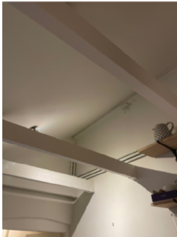
7. Photo of existing joists and lighting
