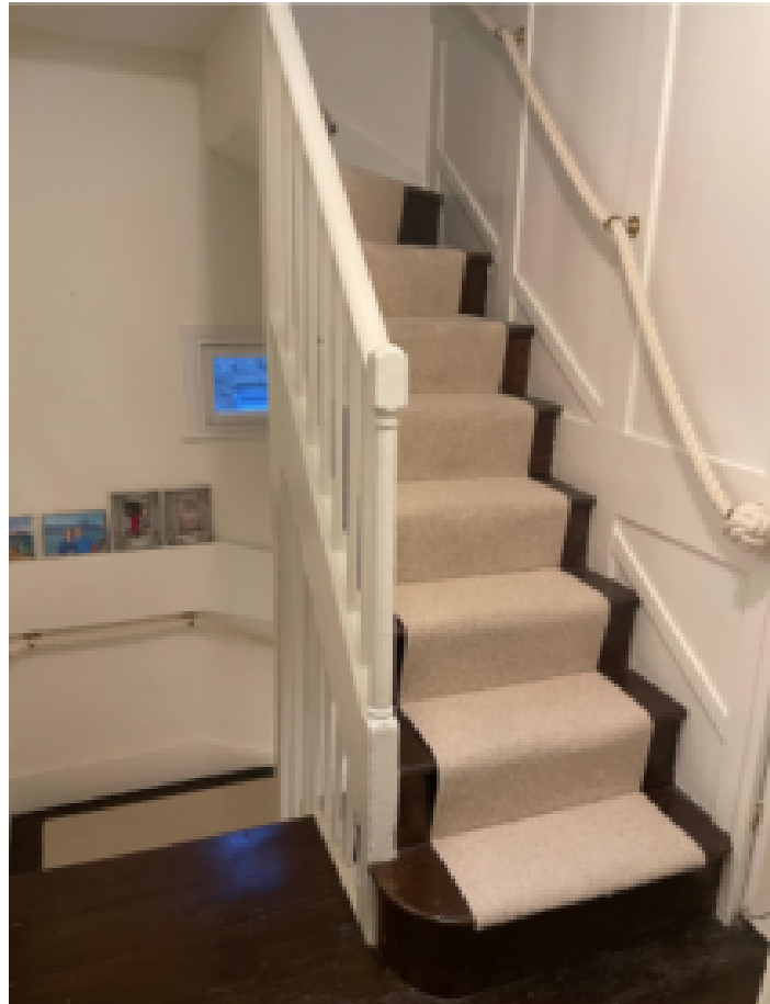
8. Photo of existing rope handrail
