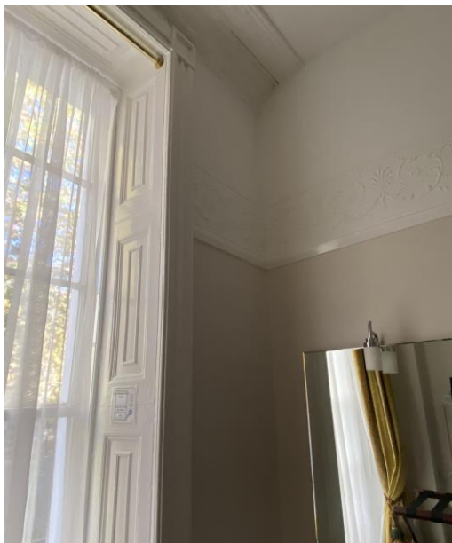
Figure 18: First floor front room to no.50 showing window architrave, shutters and cornicing architraves and cornicing surviving.
