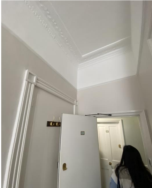
Figure 17: First floor rear to no. 49 showing a typical example of historic features of interest such as door architraves and cornicing surviving around modern partitions.
