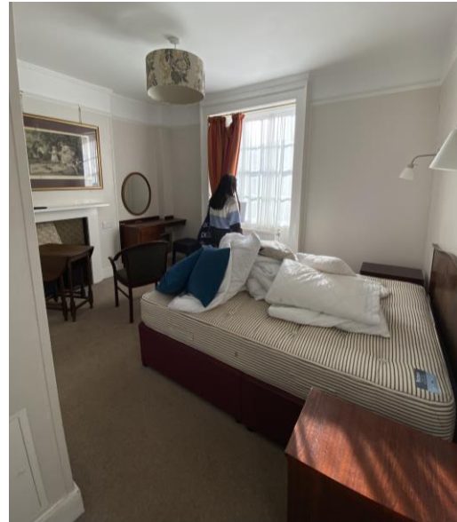
Figure 19: Second floor rear room to no. 50 with historic fireplace, skirting and cornice features. The foreground partition to the left of the image is the ensuite bathroom inserted in the room.
