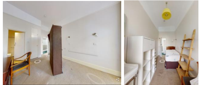
Figure 24: First floor front room of no. 49 looking toward the rear. The former room divided by modern plasterboard partitions into multiple rooms (corridor with 2 hotel rooms) The larger room (left image) contains an ensuite.
