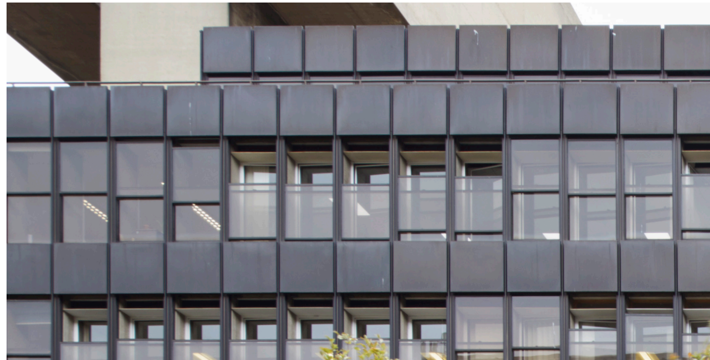
Existing aluminium glazed facade
