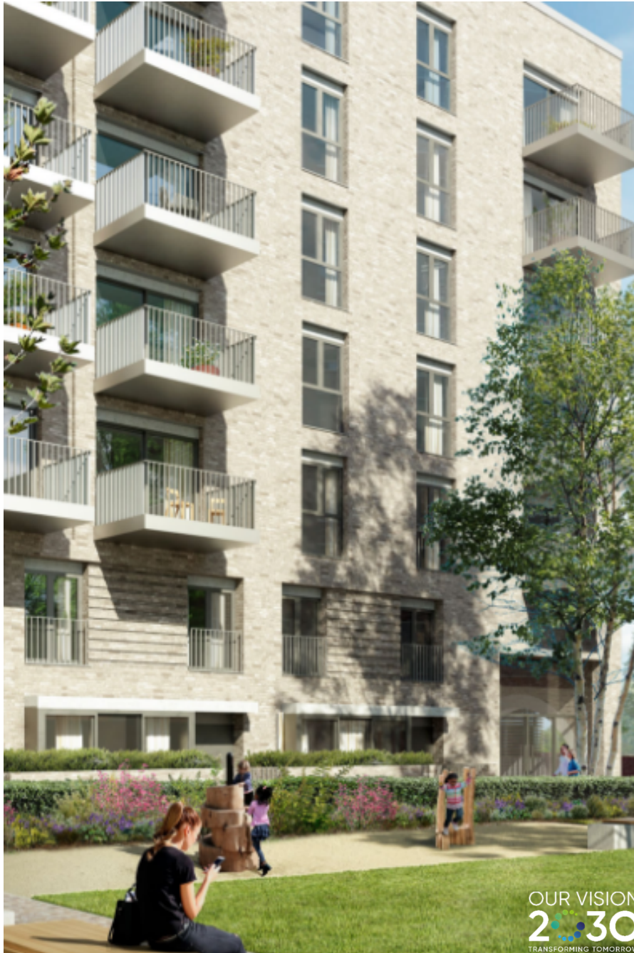
Image of Building B From DAS
