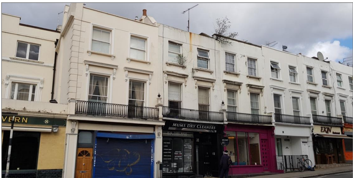
Figure 5: View of the application site in context with the neighbouring terraced properties
