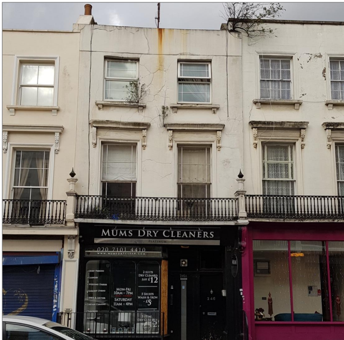
Figure 6: Front elevation of 246 Belsize Road
