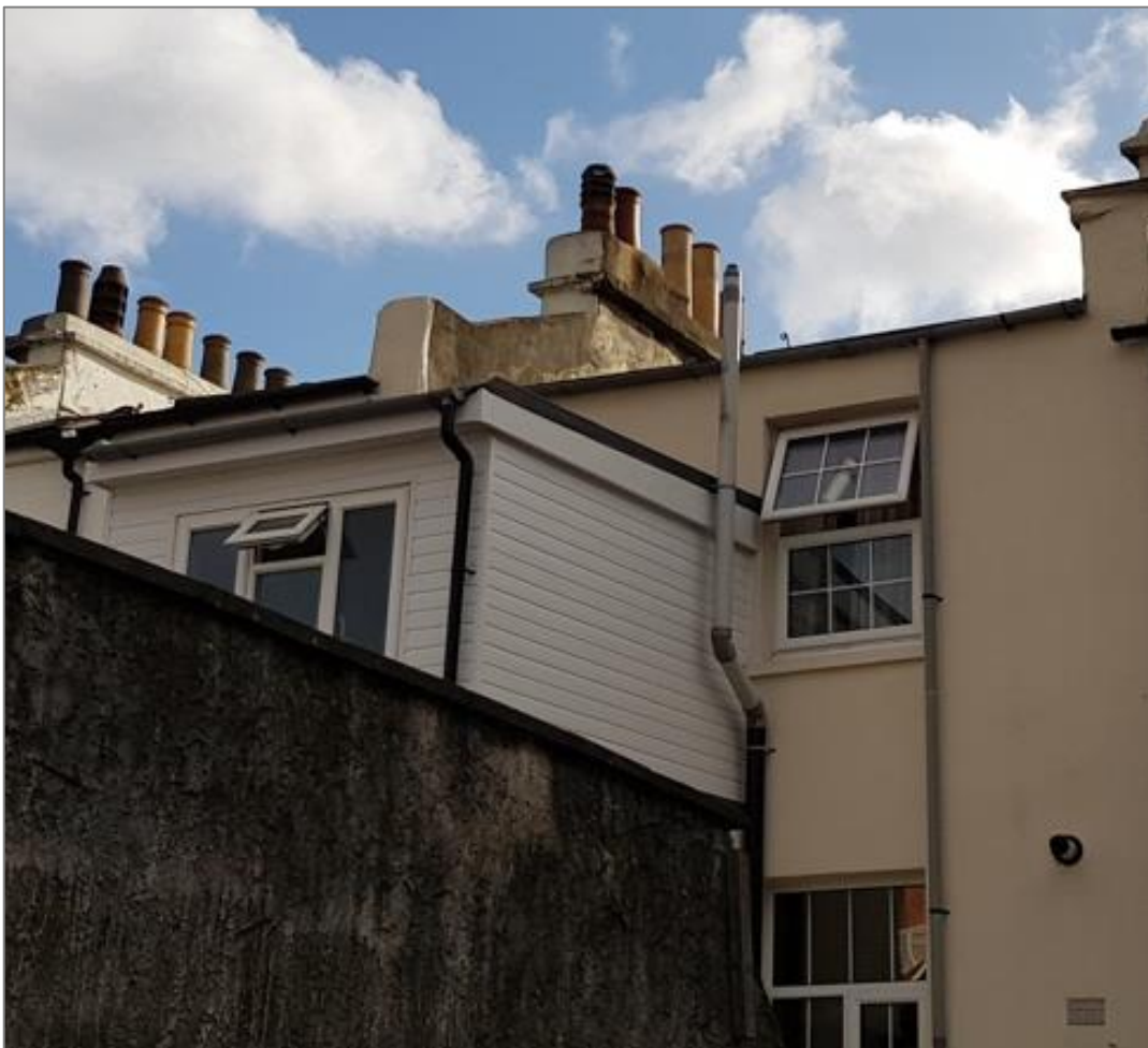
Figure 11: Existing rear outshoot with flat roof
