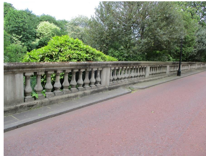
General View from Road Side of Balustrade
