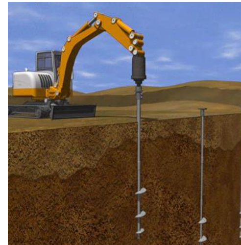
Visualisation of Excavator Installing Screw Piles
