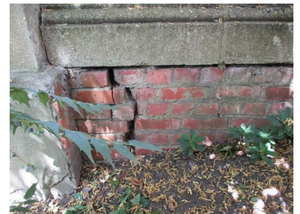
Typical Photo of Brick Retaining Wall Showing Signs of Movement
