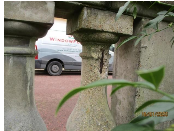
Typical Photo of Balustrade Spalling
