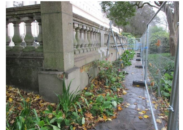
Typical Photo of Balustrade with Scaffold Support and Protective Fencing
