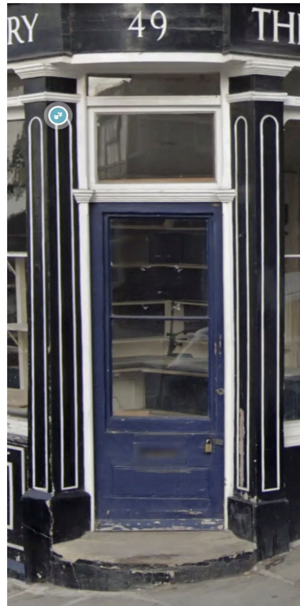
Photo of existing door to be replaced by DG.02
