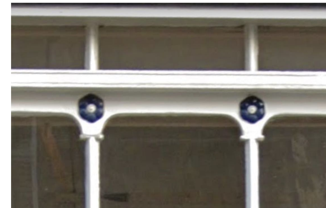
Detail 01 Original decorative flower detail to be retained and re-used in new window
