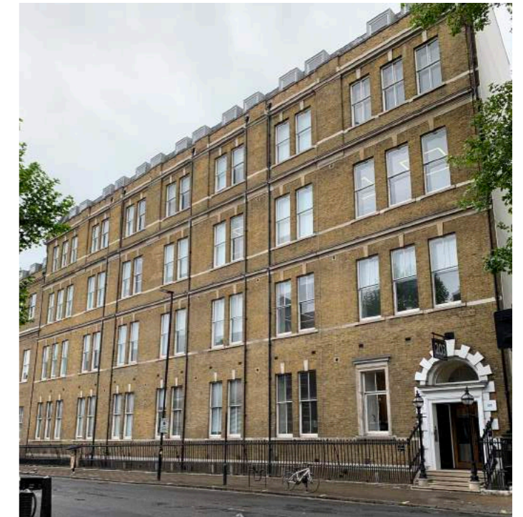
Figure 4.3 203 Eversholt, showing early 20th Century windows
