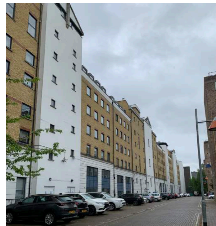
Figure 4.4 Entirely modern windows to the rear
