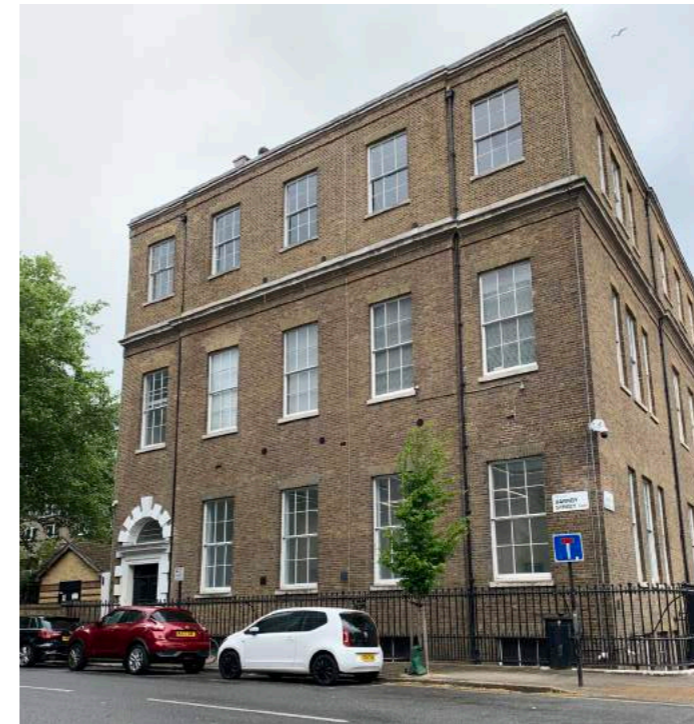
Figure 4.2 South elevation of 163 showing earliest phase of windows
