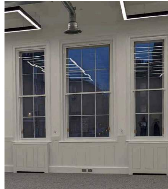
Figure 5.3 Example of existing secondary glazing applied to 163 ground floor
