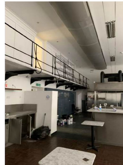
Figure 3.17 Office space used as a kitchen. Historic mezzanine in situ.
