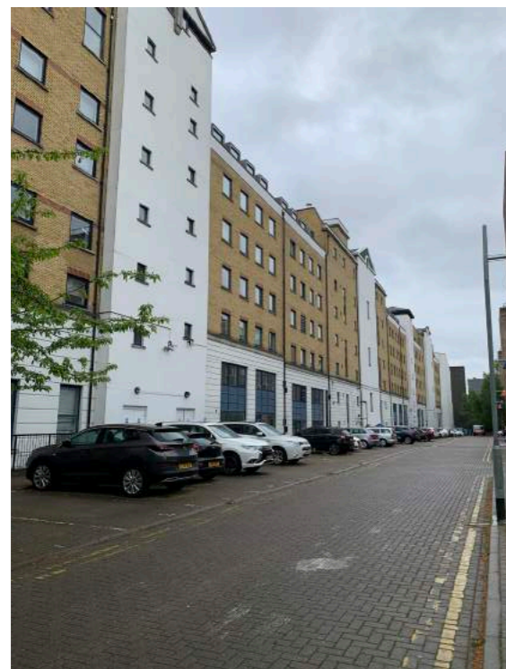
Figure 3.19 Rear elevation. View looking from the north
