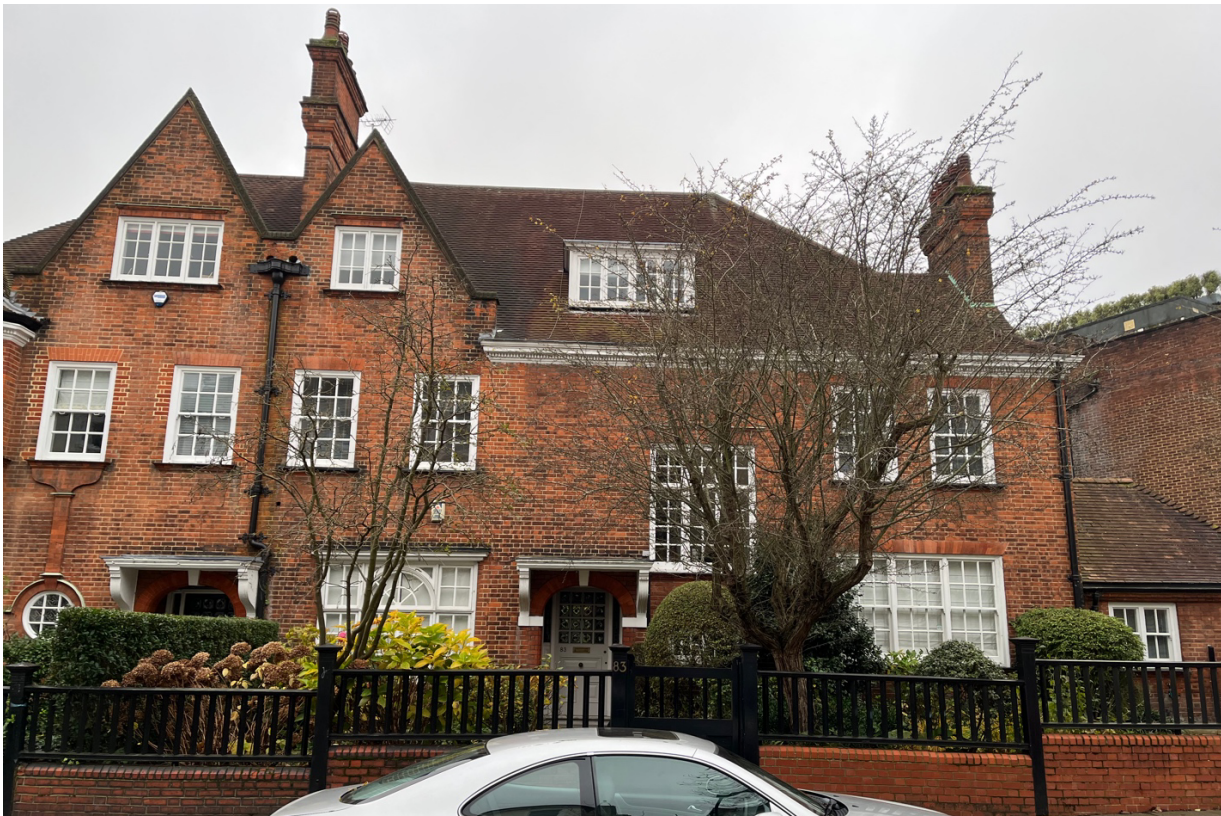
Photo 1 – Belsize Park Gardens street elevation
